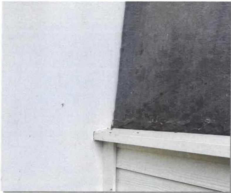
Pl. 1 Photograph showing samples of existing finishes on the main house to be incorporated on the proposed extension, including Burlington natural roofing slate (as existing) and Hardieplank and rendered walls.
