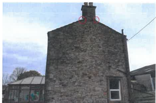
Gaps behind flashing on southern gable
