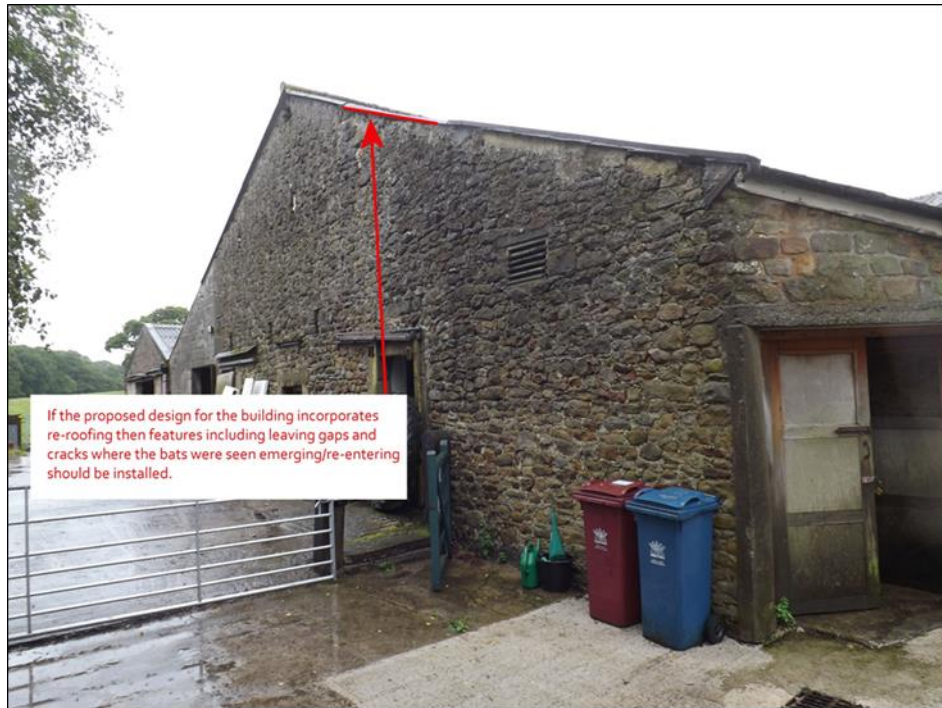
Plate 26: Narrow crevice features should be re-created for bats on the north west gable.
