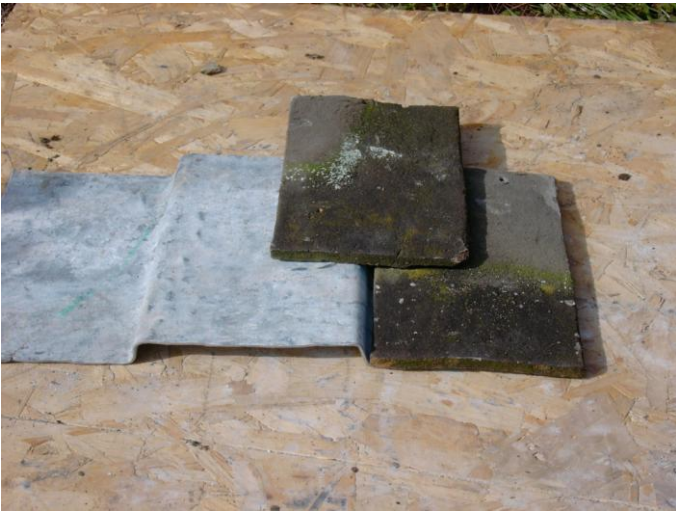
7) The completed Bat-slate alongside two tiles, showing how it'll look once fitted.
