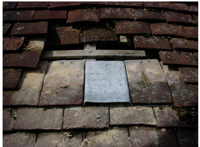
10) Tiles are refitted around the Bat-slate.
