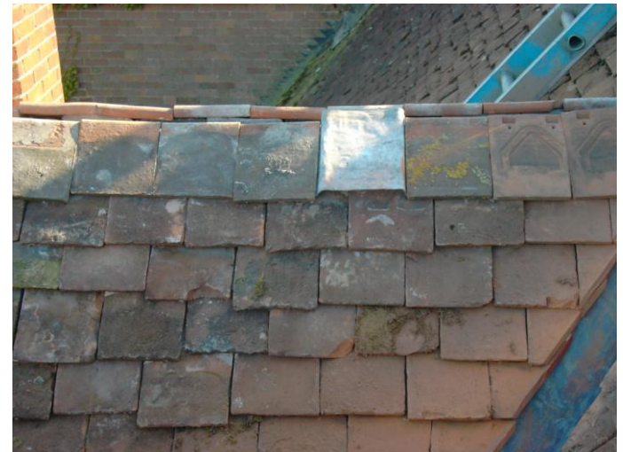
16) The Bat-slate can also be fitted by replacing one of the shorter eave tiles. The Bat-slate should be cut accordingly.
