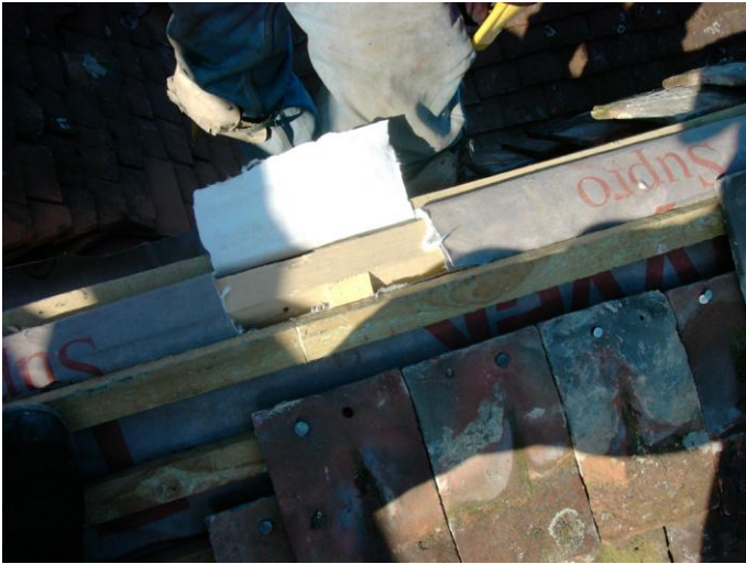
13) This picture shows a hole being cut in the roofing felt when the Bat-slate is fitted in/near the ridge tiles. This will allow bats access into the loft/attic area.
