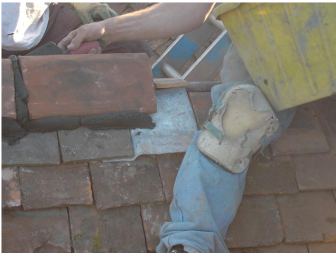
17) This picture shows the ridge tiles being bedded on. If the mortar joint in the ridge tiles come 'above' the Bat-slate, material like a broken tile should be placed on the Bat-slate to avoid the mortar blocking bat access.
