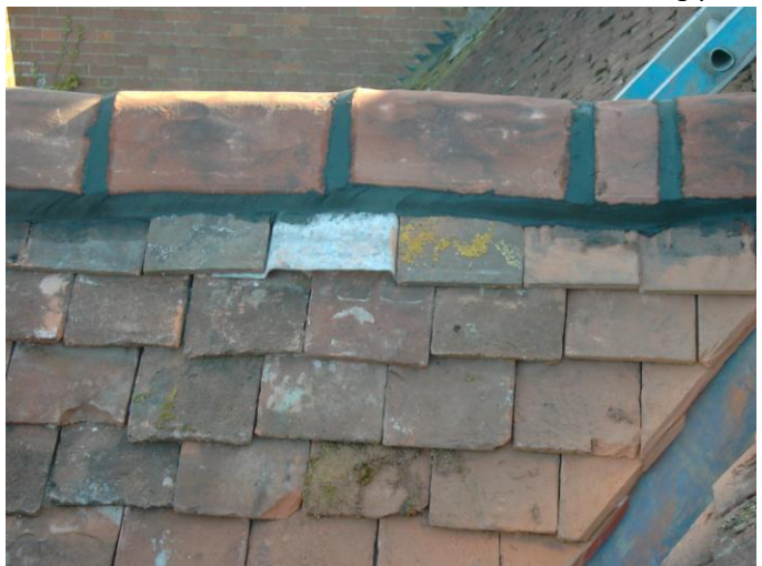
18) Ridge-line showing the Bat-slate in place of the top eave tile.
