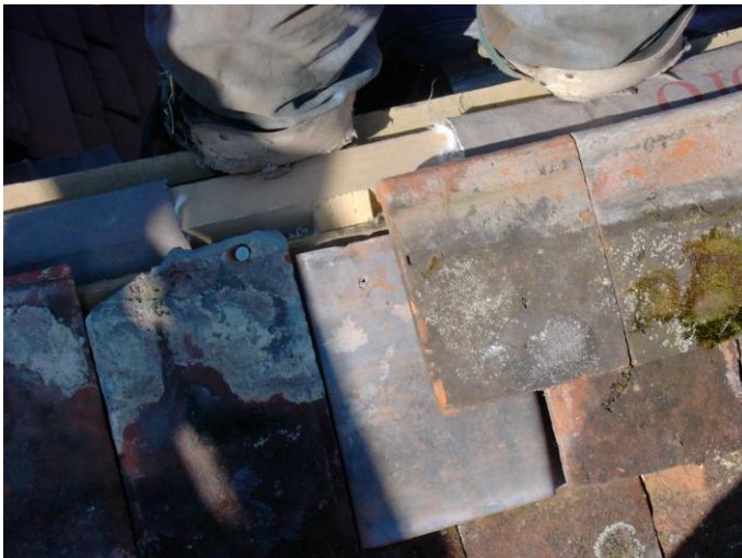
15) The top 'eave' tiles are fitted in the normal way.
