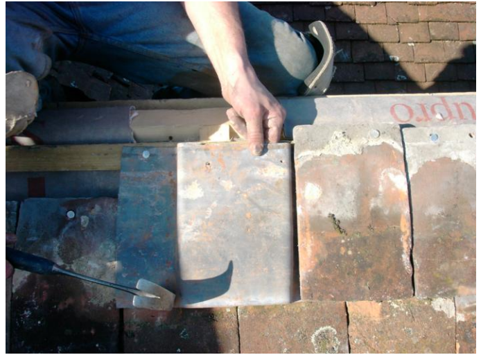
14) The Bat-slate is fitted in the same way as the previous one, being the same length and width as a plain tile and nailed twice into the top batten. Note the Bat-slate is above the hole in the felt.
