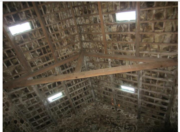
Photo 10: Underside of roof at attached barn showing roof lights
