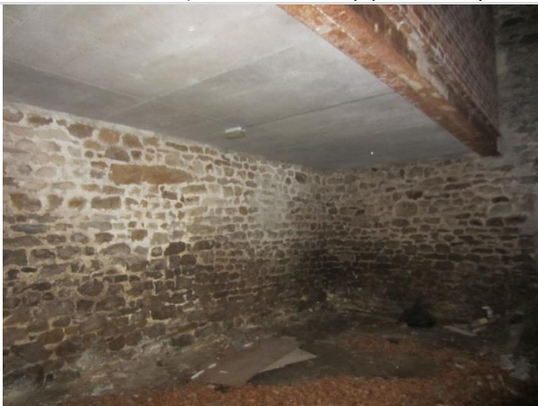
Photo 9: Interior of attached barn
