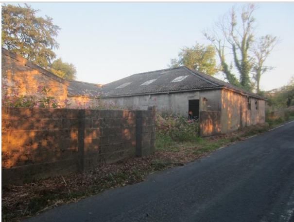
Photo 11: Southern and eastern elevations of the shippon
