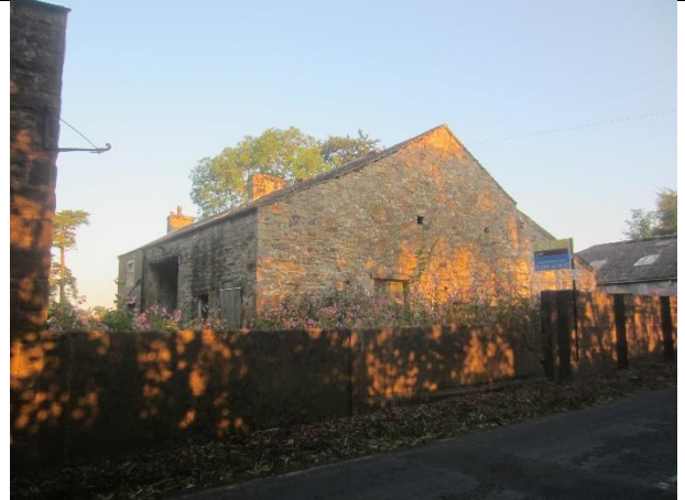
Photo 8: Eastern elevation of attached barn
