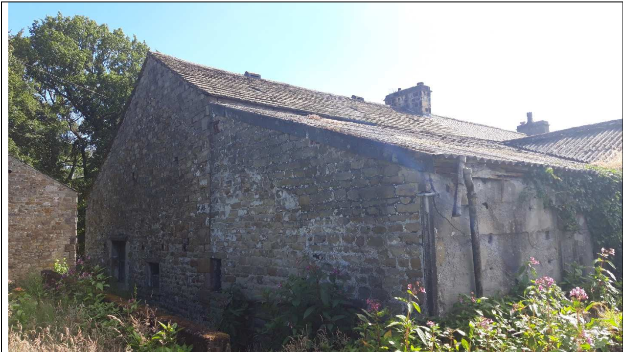
East Wall of North West Barn
