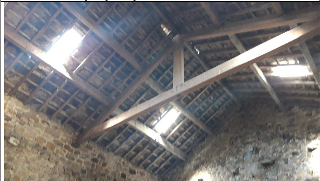
Roof Over North West Barn
