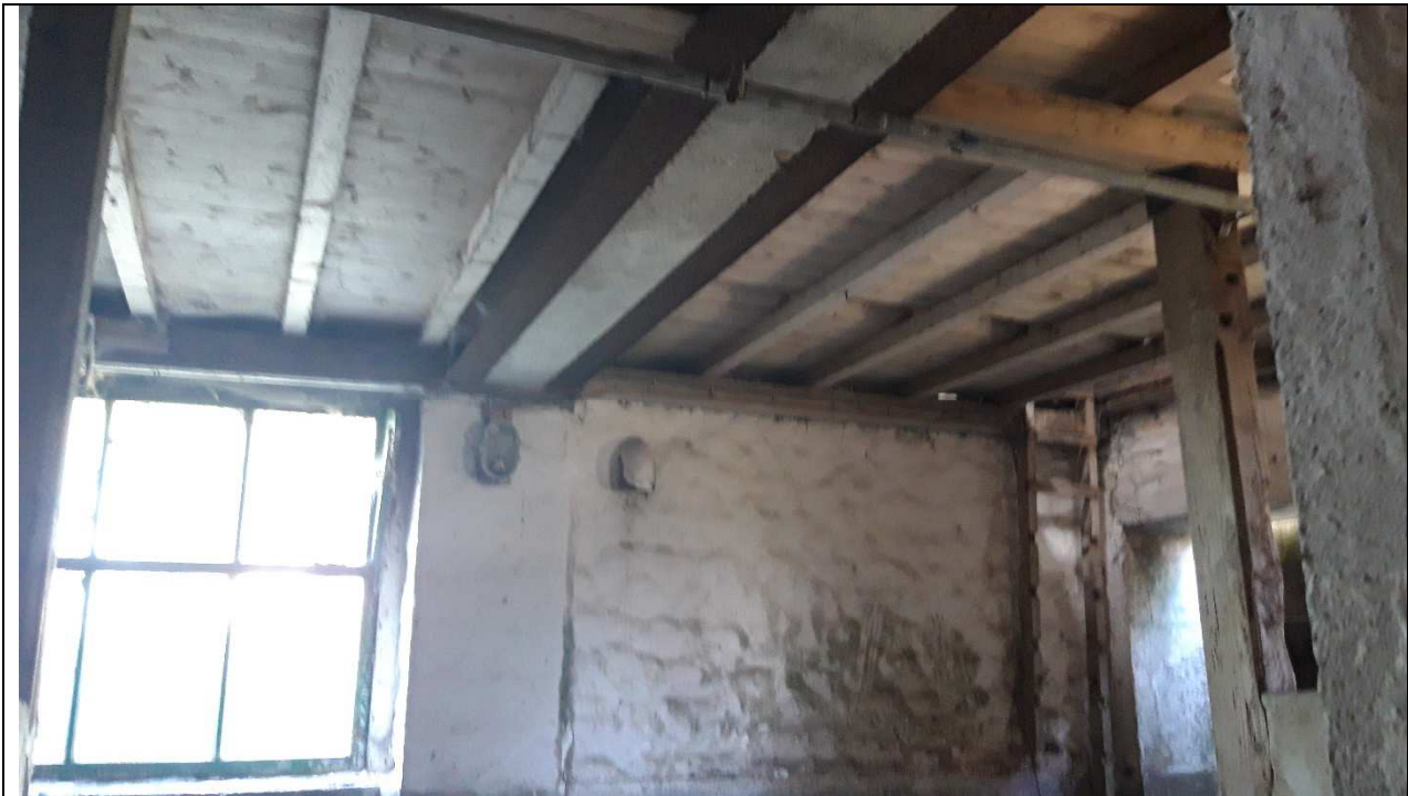
Lightweight Ceiling Over East Side of North West Barn
