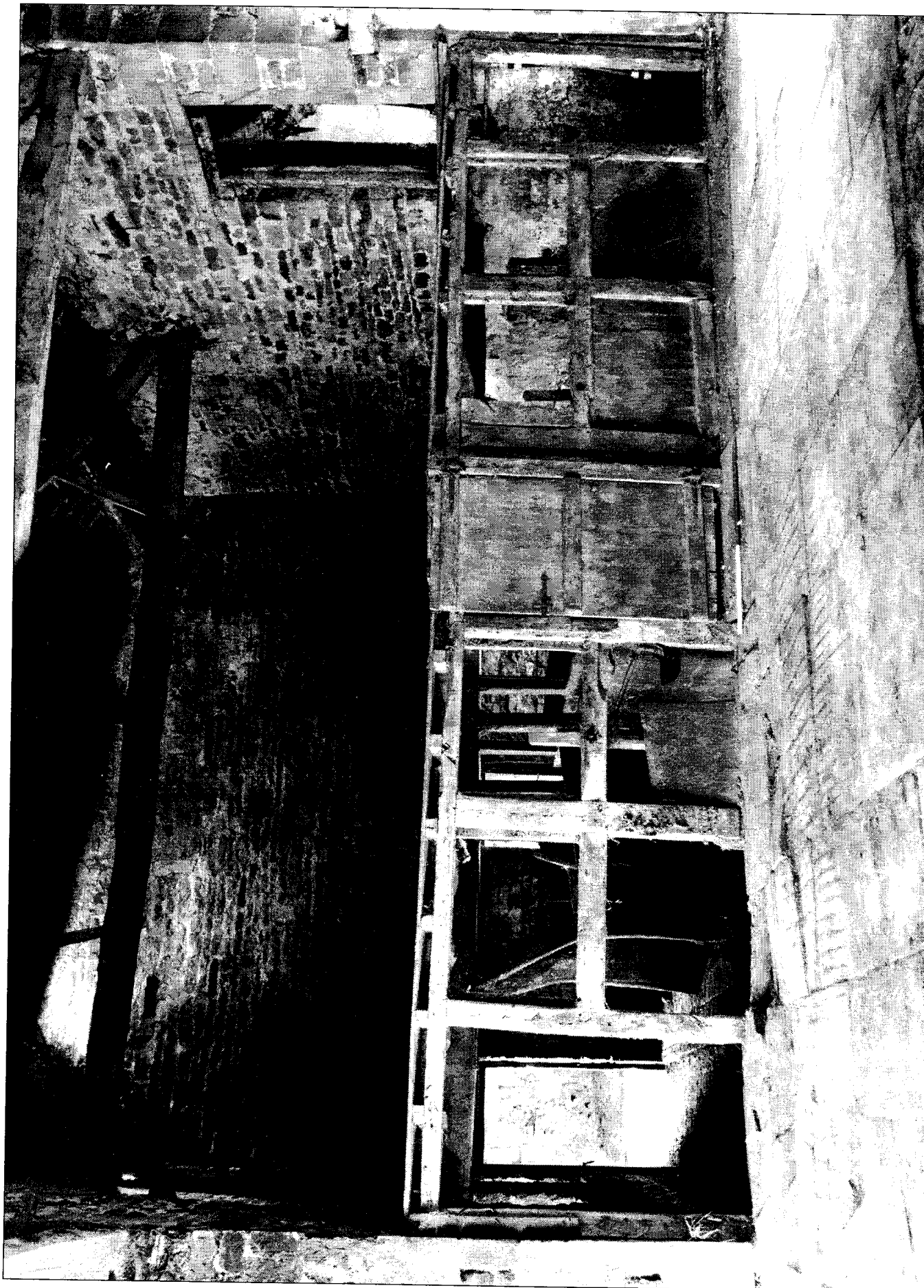
Photo 26: Interior of barn, showing threshing floor and timber-framed shippon with hay loft over, from the north-east
