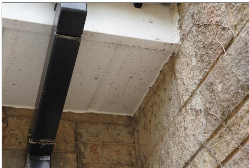
Photo 4: Well-sealed uPVC soffit boxes.
