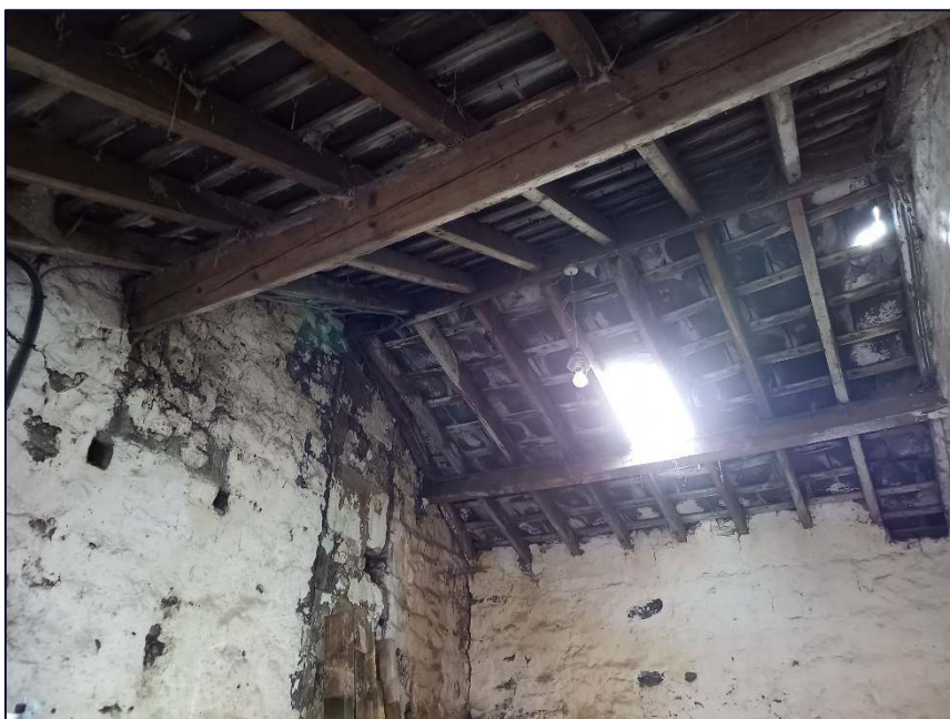
Plate 16: Detail of roof structure in Building A
