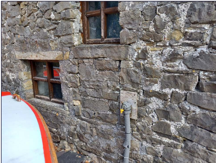
Plate 24: Blocked window, south-west elevation of Building B
