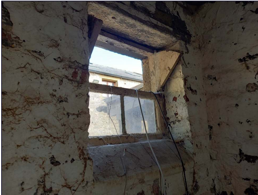
Plate 15: Detail of one of the windows with upper section that opened inwards (Building A)
