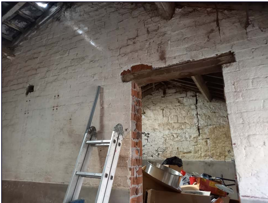
Plate 14: Internal brick wall which divides Building A into two rooms
