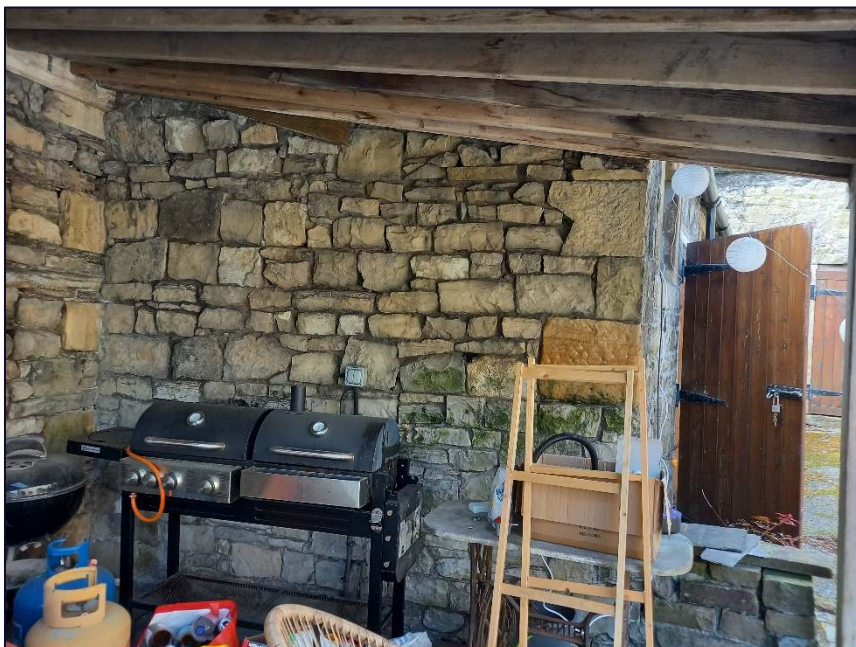
Plate 10: North-east elevation of Building A
