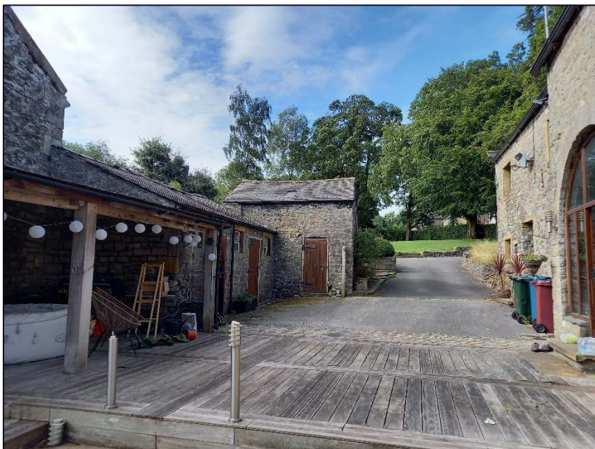
Plate 4: View looking west showing Crow Trees Barn to right of photograph, and the buildings proposed for conversion to left of photograph
