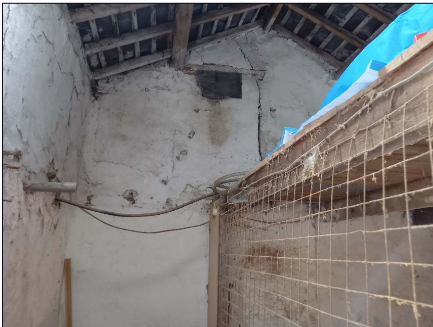
Plate 26: View looking south showing the interior of Building B
