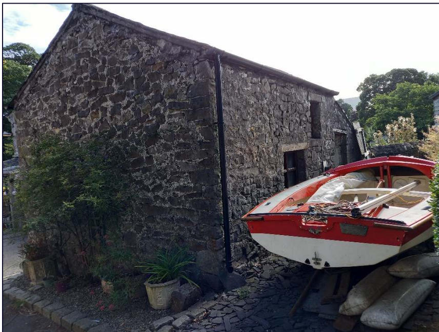
Plate 22: North-west gable and south-west elevation of Building B
