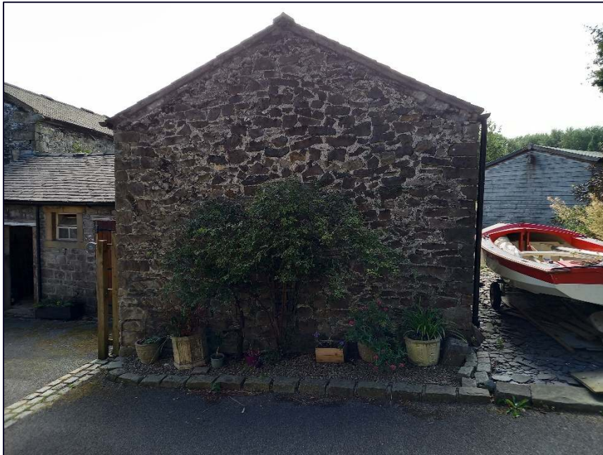
Plate 21: North-west gable of Building B
