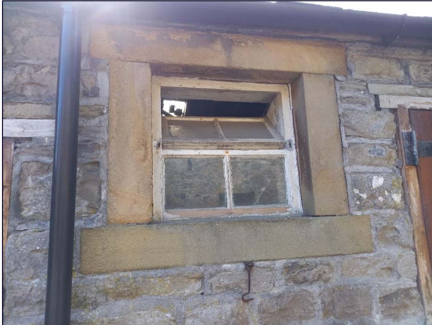
Plate 9: Detail of window, north-west elevation of Building A
