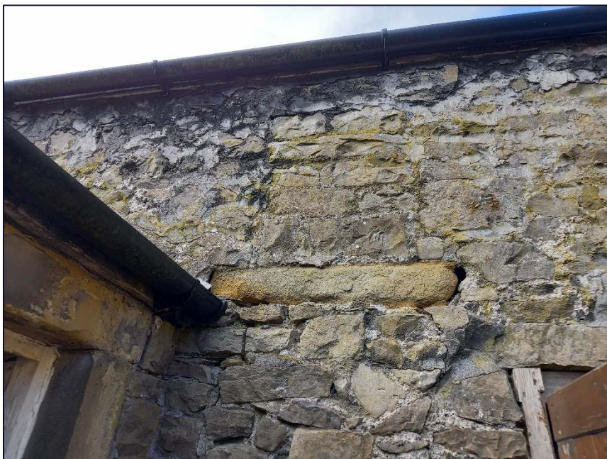
Plate 20: Detail of blocked window, north-east elevation of Building B
