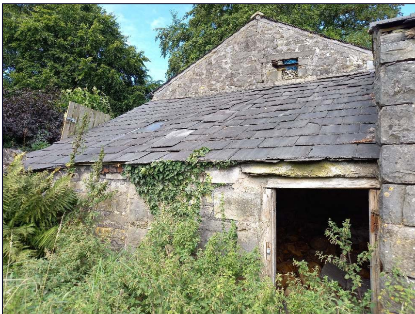
Plate 30: South-east elevation of Building C
