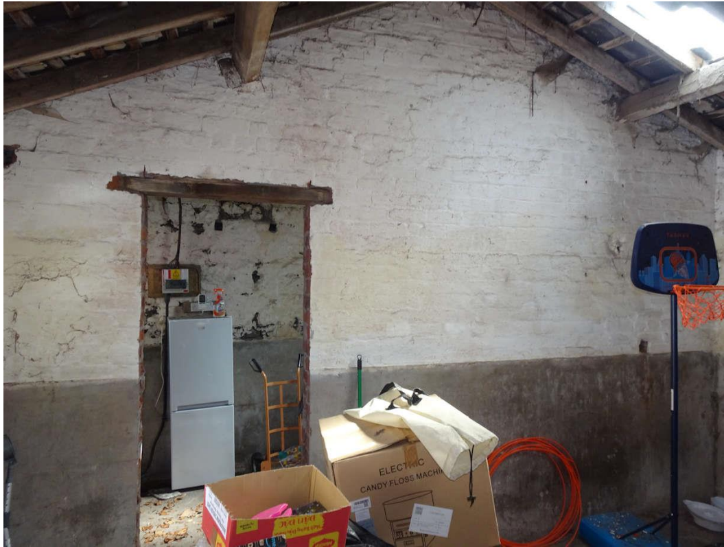
Photograph 35: Sitting Room / Dining Room Left Partition
