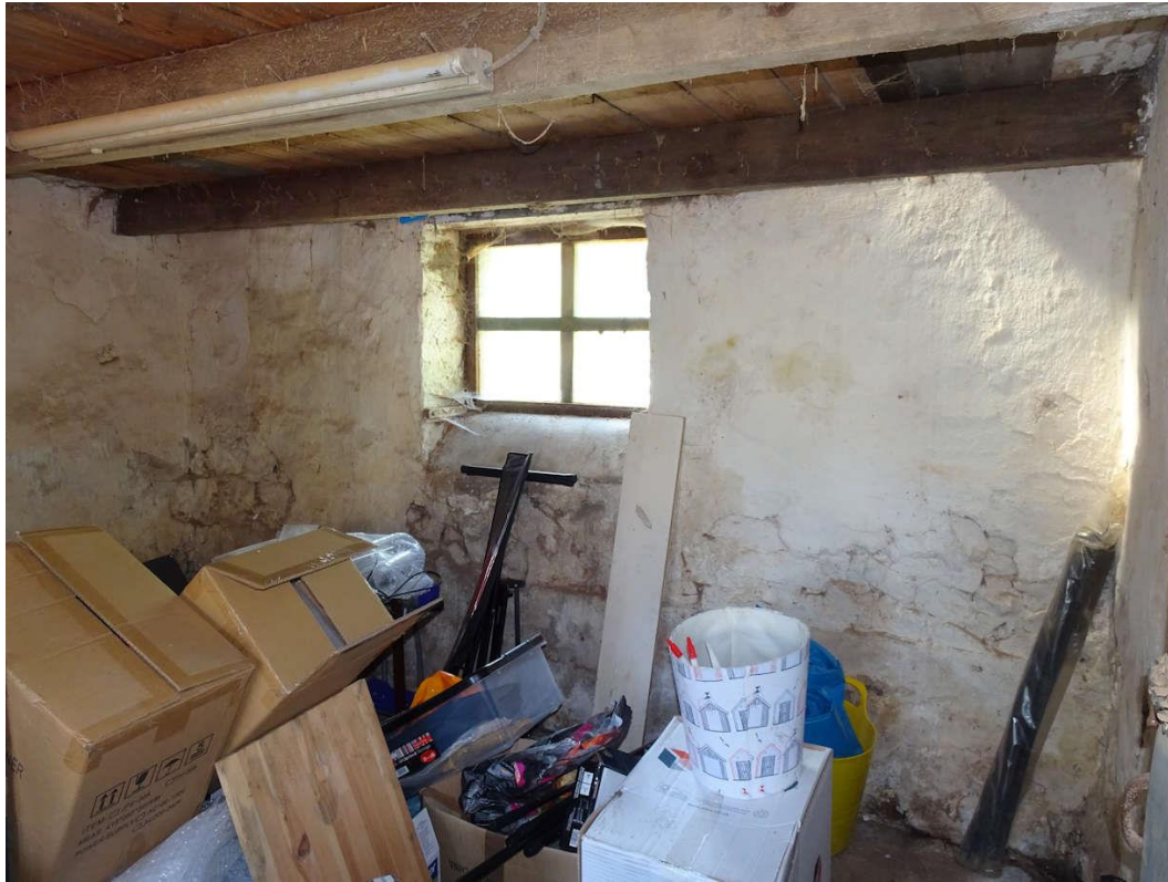
Photograph 25: Bedroom Right Side Elevation
