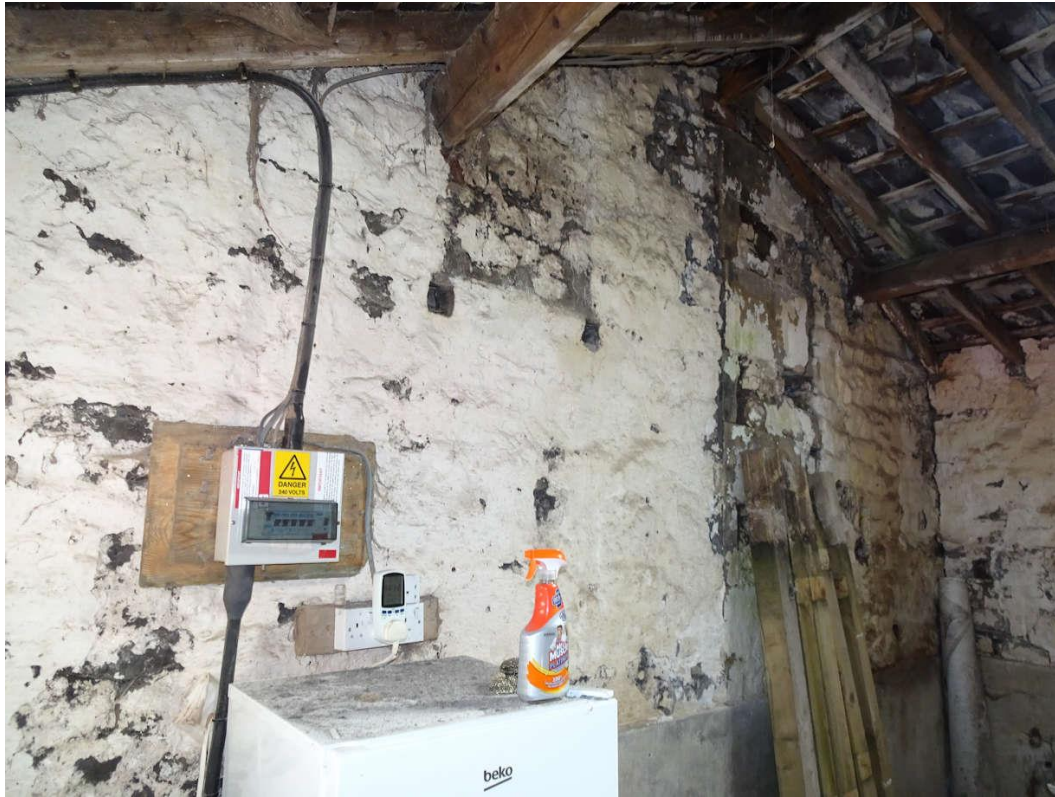
Photograph 41: Kitchen / Utility Room Left Elevation
