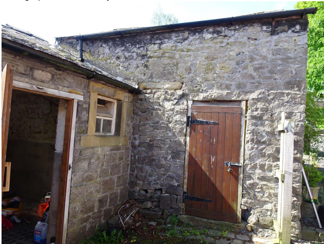
Photograph 8: Bedroom Left Side Elevation
