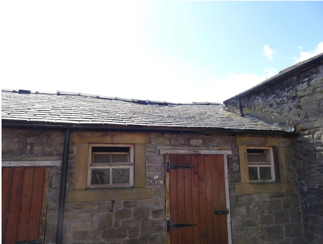
Photograph 21: Dining Room Roof Canopy At Front
