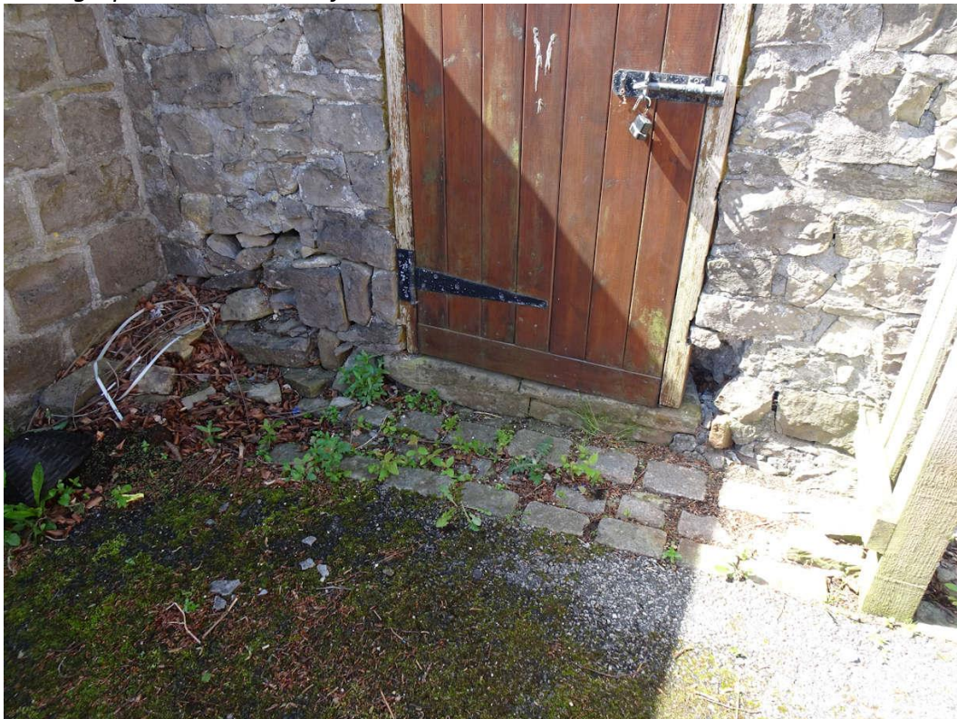
Photograph 10: Bedroom Left Side Elevation At Ground Level
