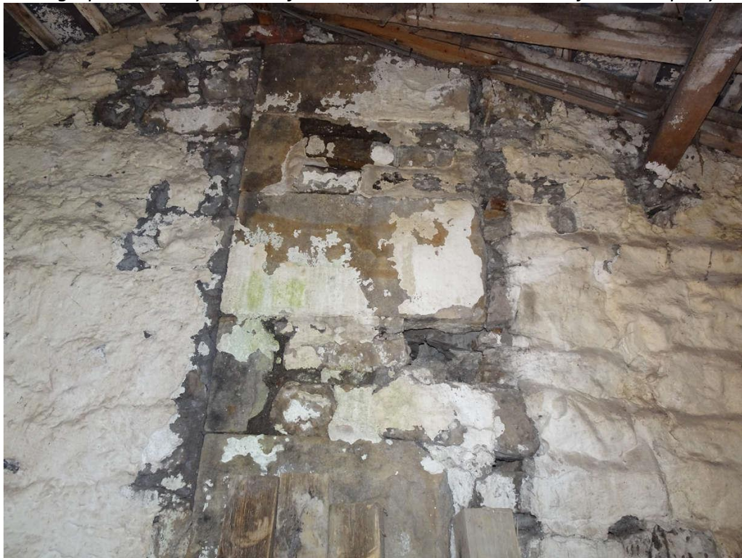
Photograph 42: Utility Room Left Elevation At Junction With Adjacent Property
