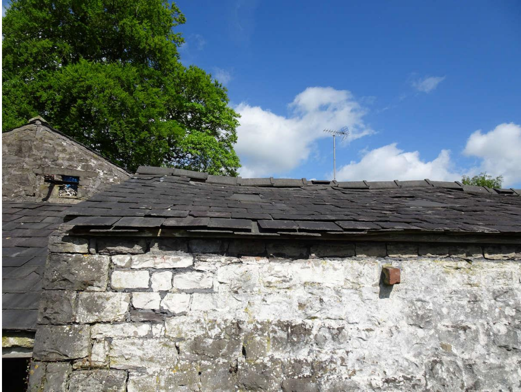
Photograph 19: Sitting Room Roof Canopy At Rear
