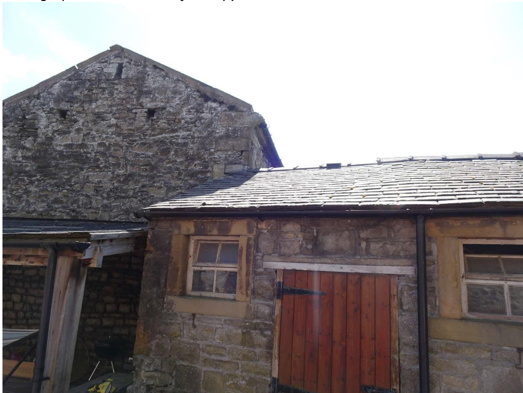
Photograph 22: Kitchen Roof Canopy At Front
