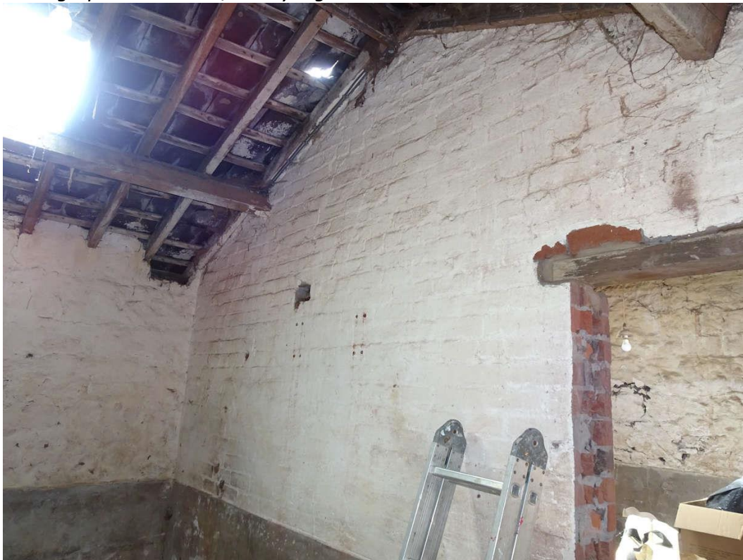
Photograph 40: Kitchen / Utility Right Partition
