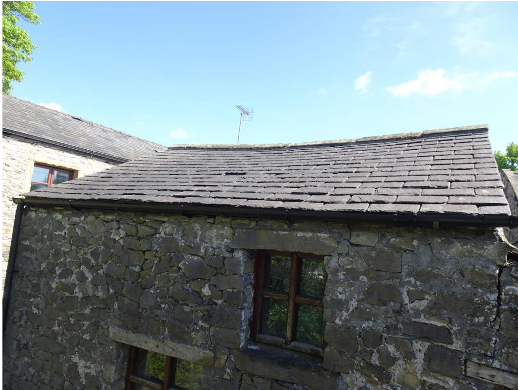
Photograph 11: Bedroom & Bathroom Roof Canopy
