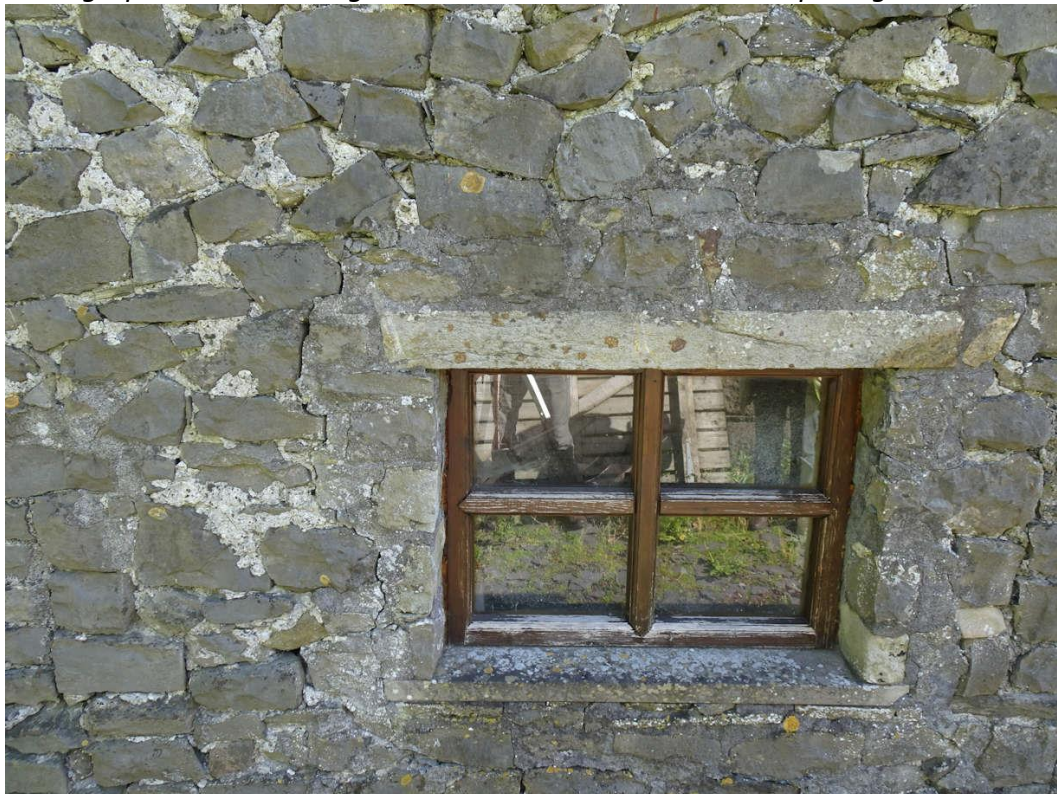
Photograph 4: Bedroom Right Side Elevation Front Window Opening
