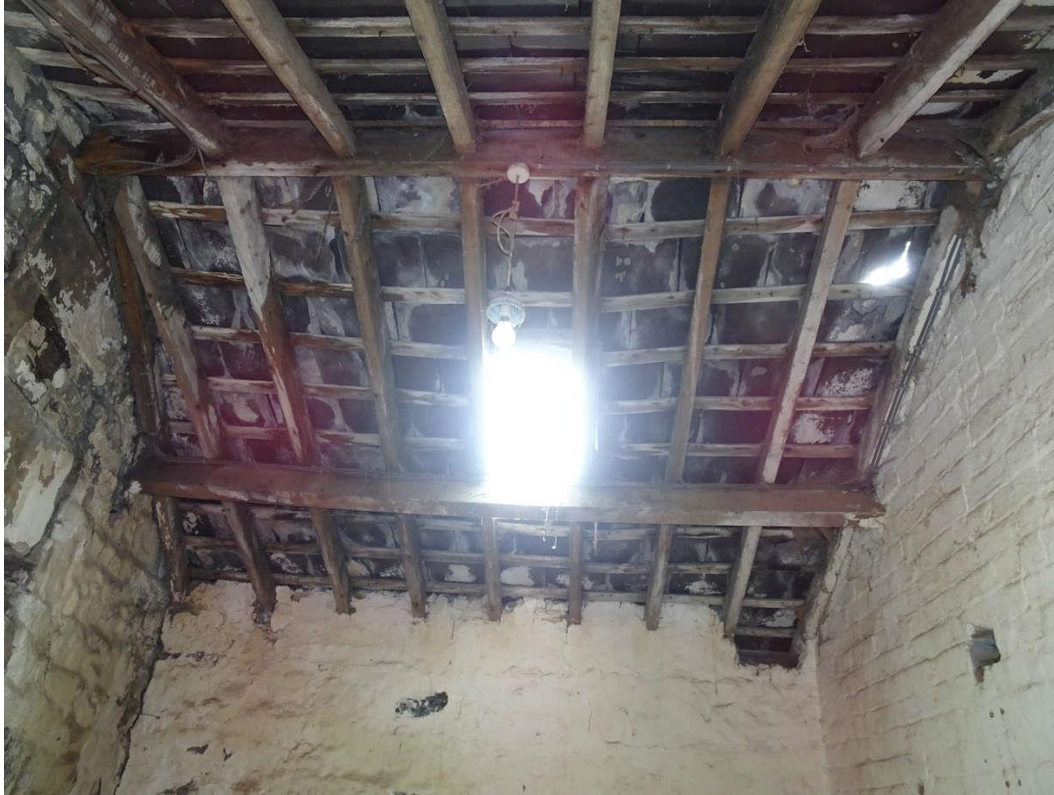
Photograph 43: Kitchen / Utility Room Roof Canopy
