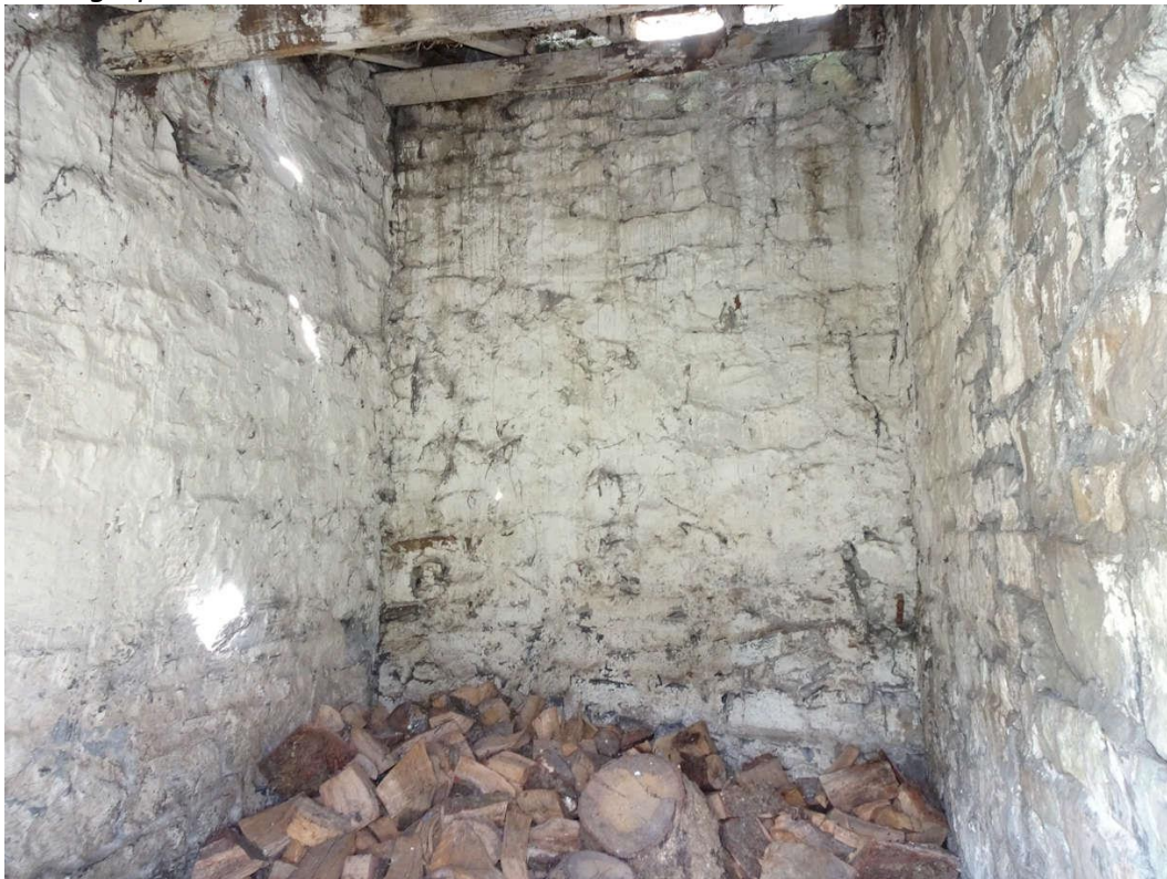
Photograph 30: Bathroom Front Partition
