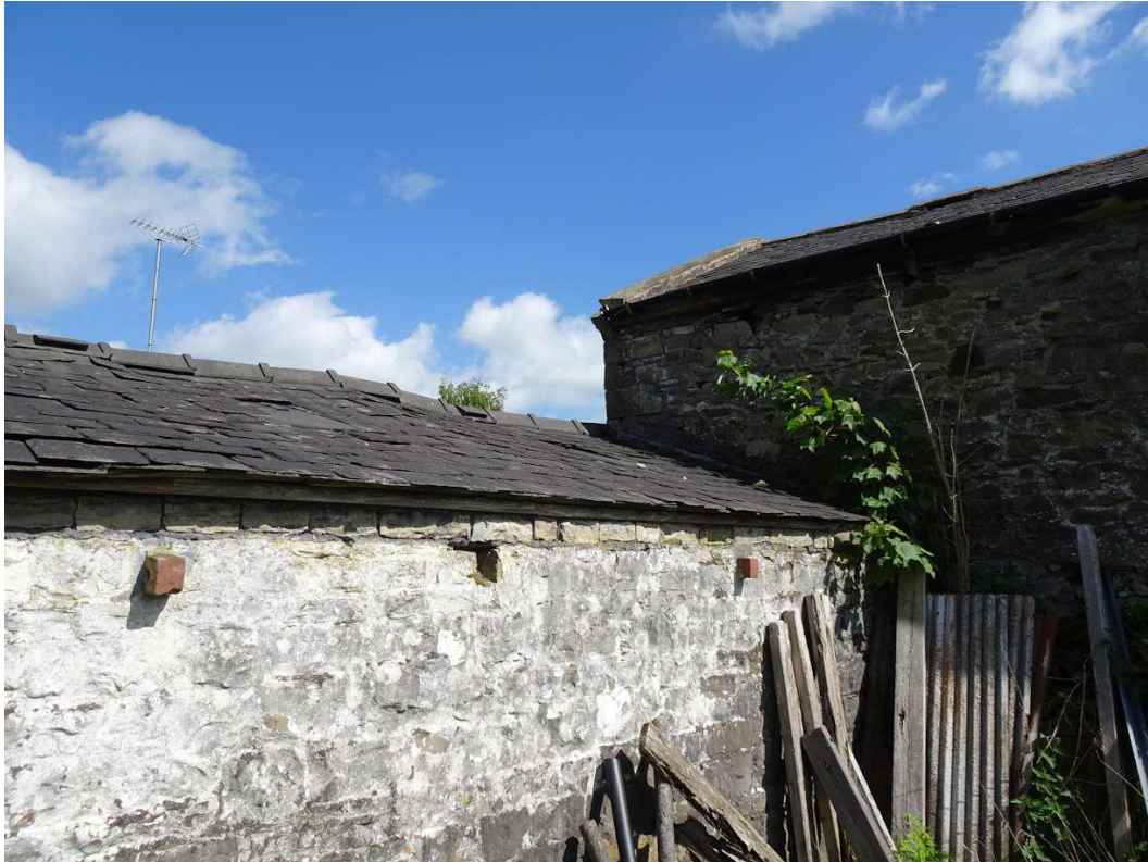
Photograph 20: Utility Room Roof Canopy At Rear
