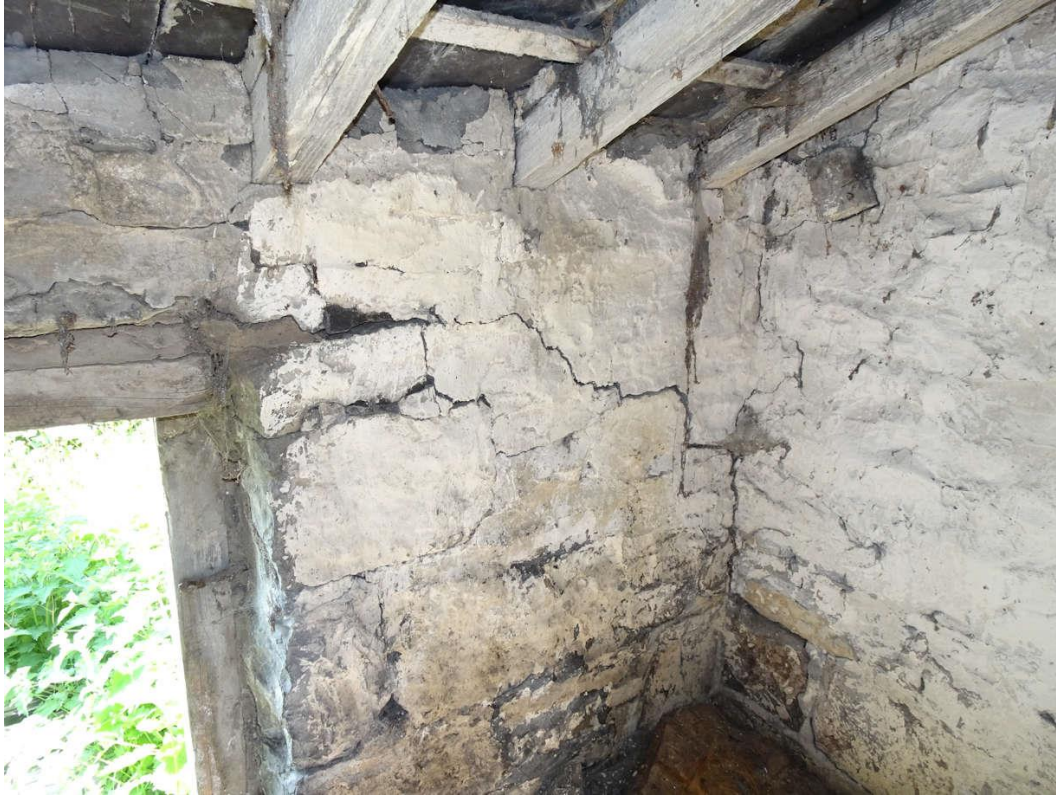
Photograph 31: Bathroom Rear Elevation
