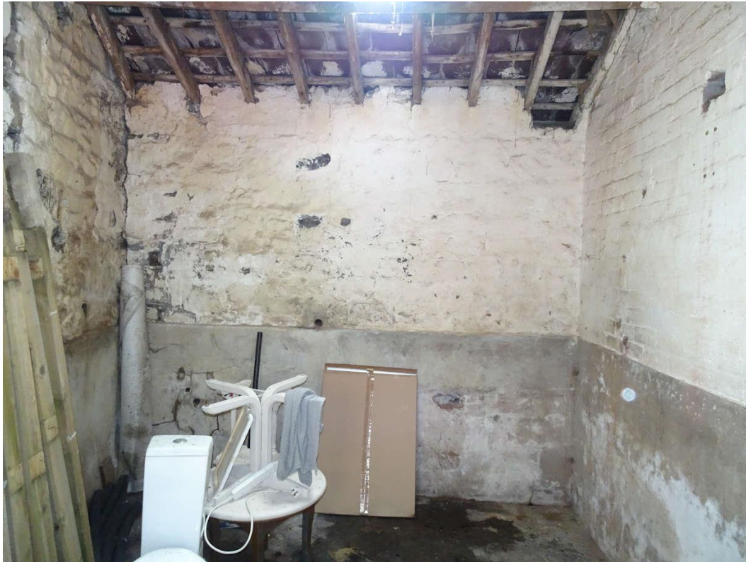
Photograph 39: Utility Room Rear Elevation
