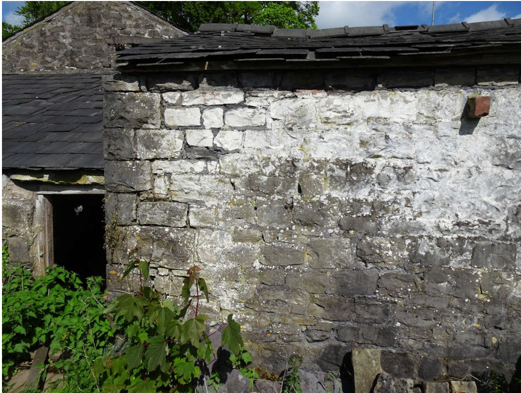
Photograph 15: Sitting Room & Utility Rear Elevation At Right
