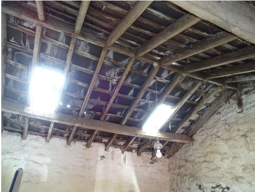
Photograph 37: Sitting Room / Dining Room Roof Canopy
