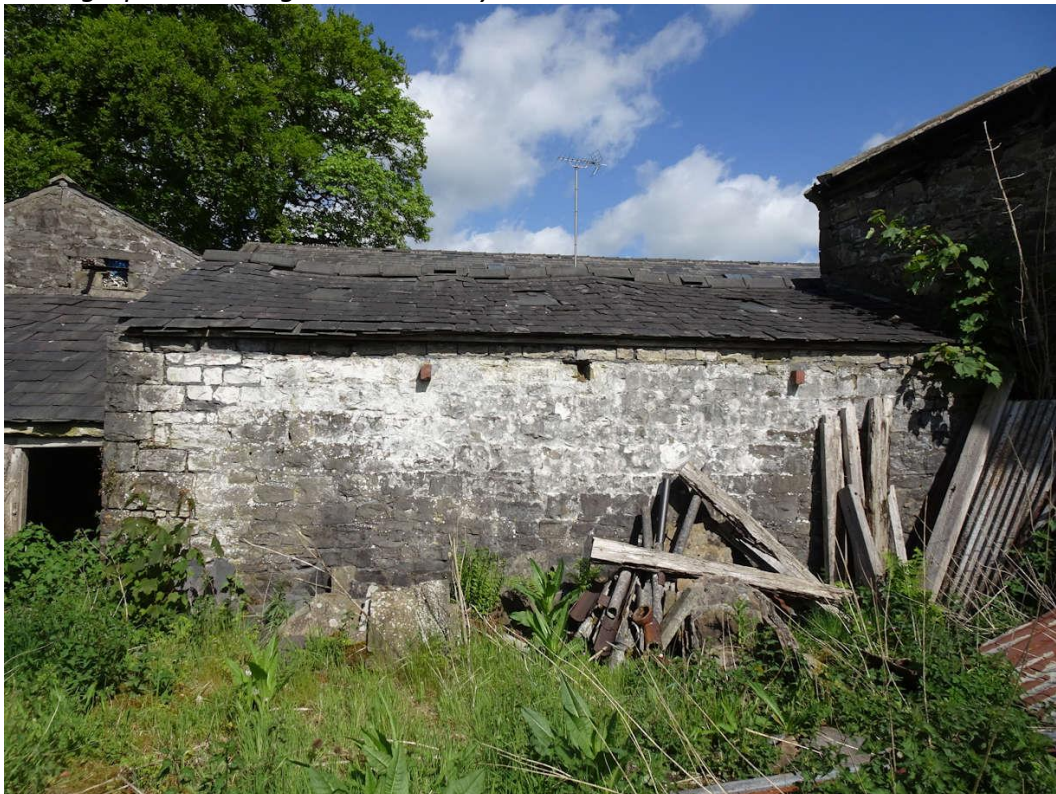
Photograph 14: Sitting Room & Utility Rear Elevation
