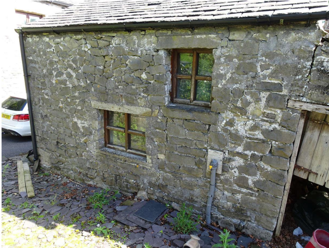
Photograph 3: Bedroom Right Side Elevation
