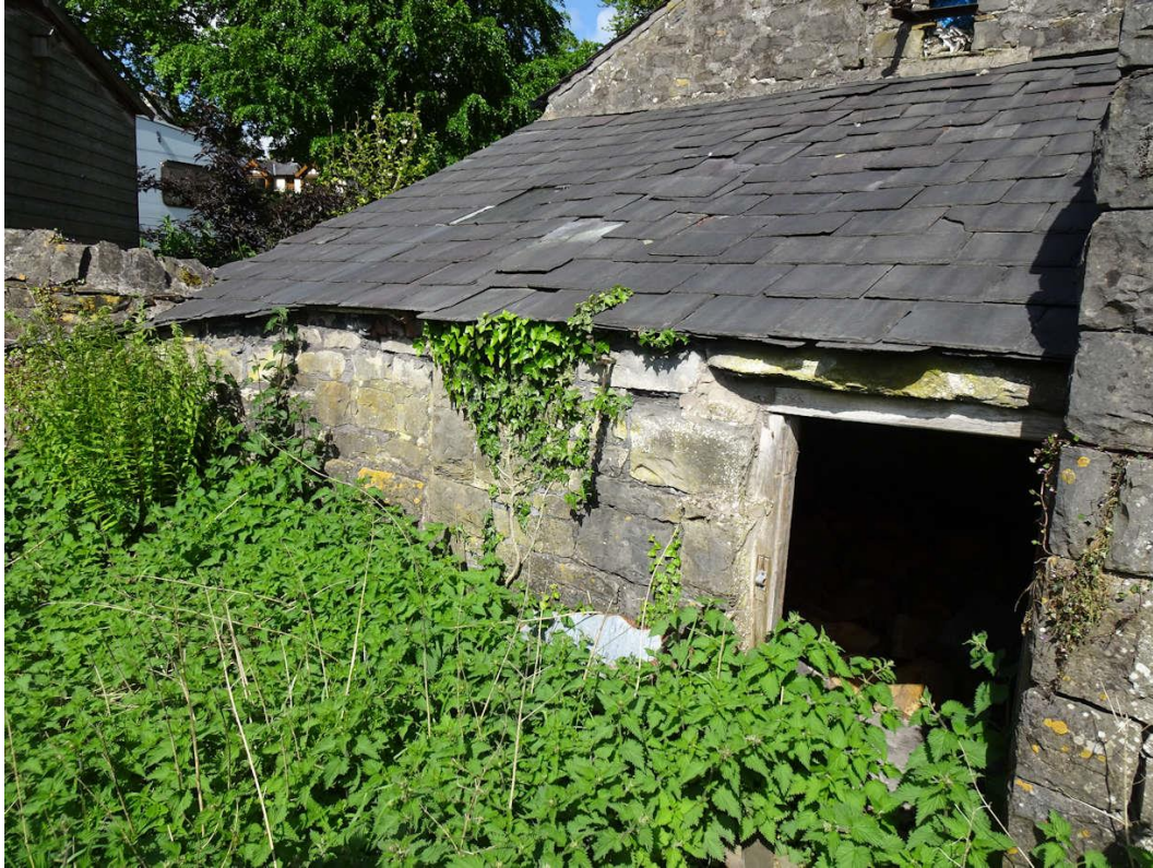
Photograph 13: Bathroom Rear Elevation & Roof Canopy
