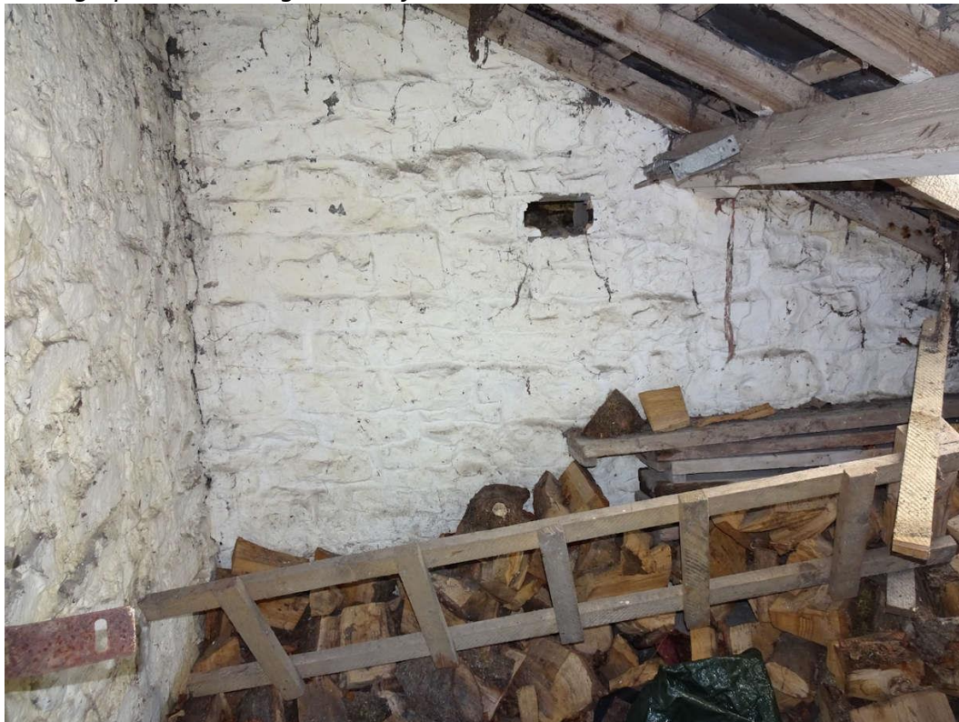
Photograph 28: Dressing Room Left Partition
