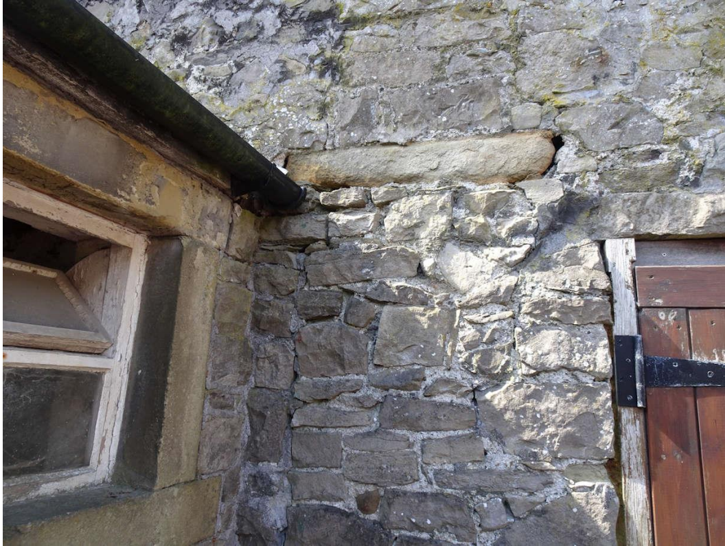
Photograph 9: Bedroom Left Side Elevation To Rear Of Doorway
