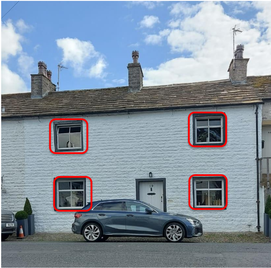
Existing front elevation showing the 4 windows to be replaced
