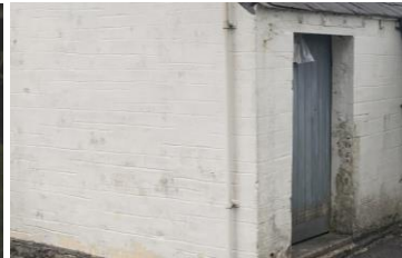
Block with render finish front section of outbuilding
