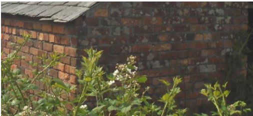
Brick rear section of outbuilding
