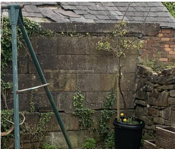
Dressed stone block walls to the garage side wall. Brick and random stone rear elevation.
