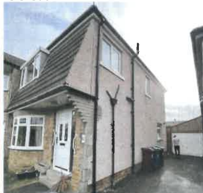
Side elevation of the house and front of Garage
