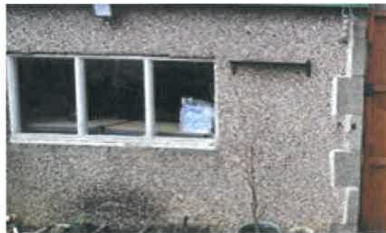
Garage side wall.
