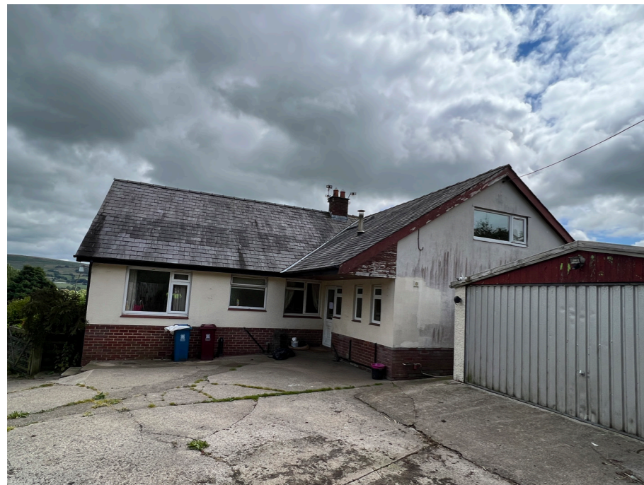
existing property - rear elevations
