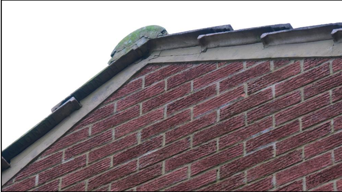
Image of west gable showing well mortared verge with no gaps
