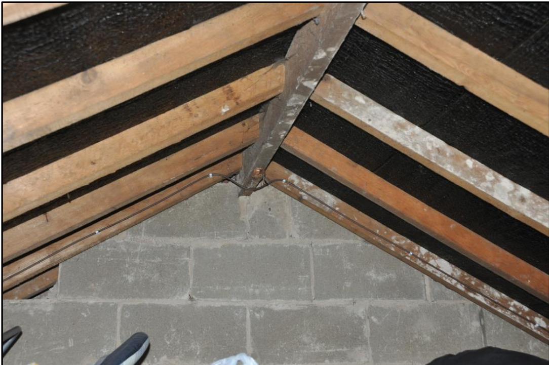
Image of roof void above showing block walls (well-sealed) and intact bitumastic roof liner
