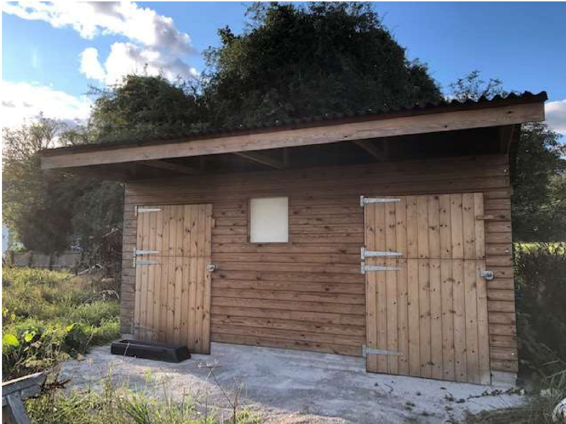
Replacement Timber Store, As Built Photo
