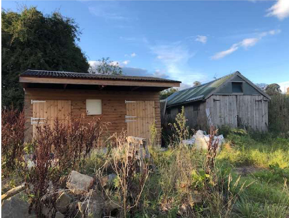
Replacement building is located on the previous position directly adjacent to an existing dilapidated timber building.
