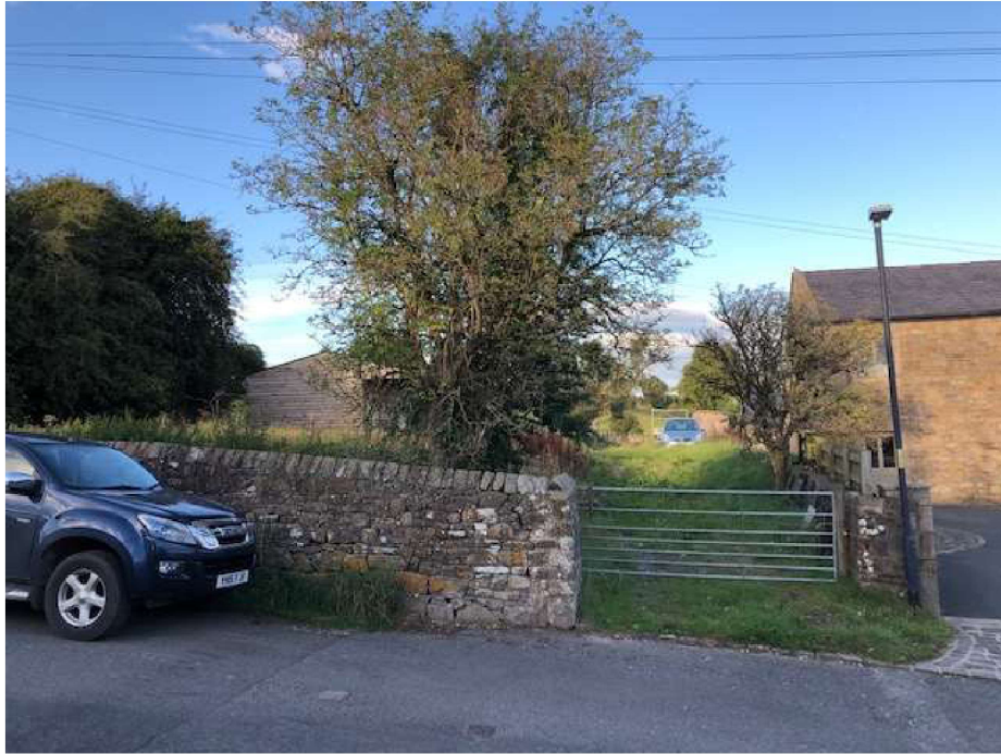
View from Back Lane, of Entrance Gate and replacement timber building in background.
