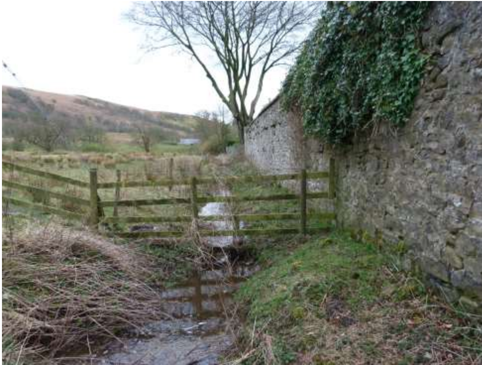
Photograph 1 – Outside northeast corner of the site looking south along boundary
