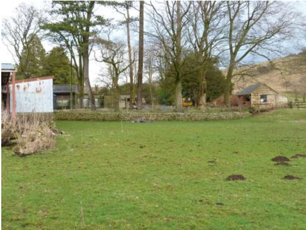
Photograph 5 – Western boundary retaining wall at development site
