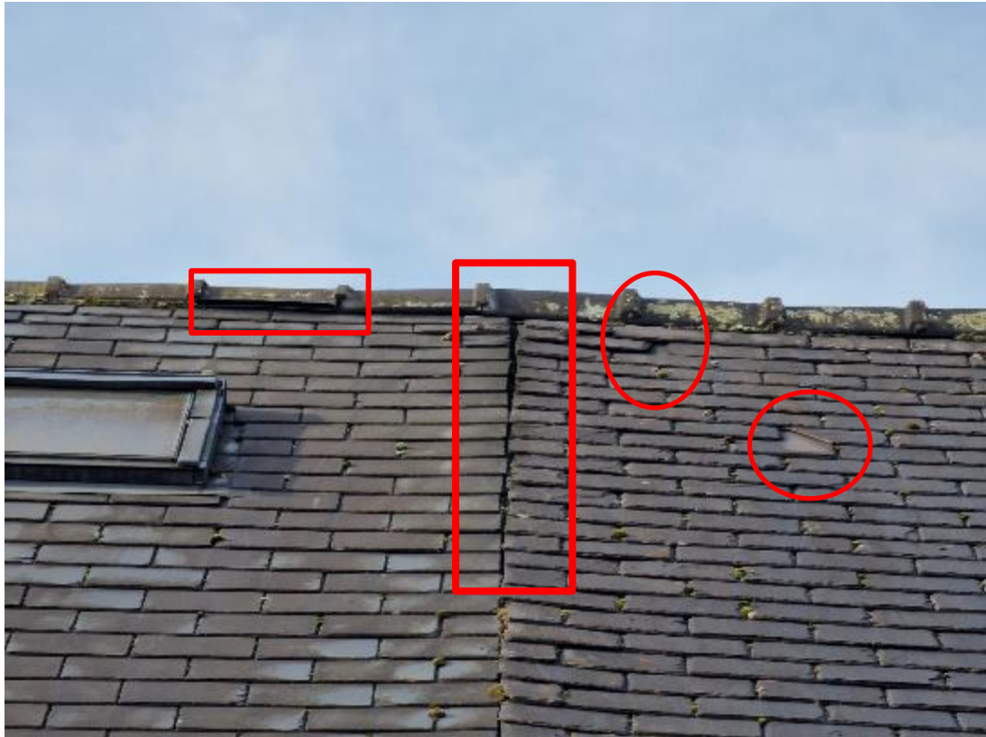
Plate 2 – A close up of the eastern elevation; see gaps in tiles acting as PRFs
