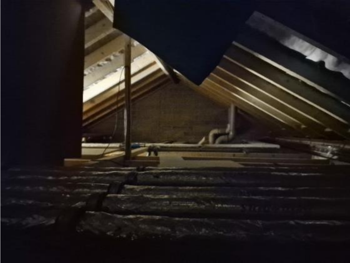
Plate 11 – General character of Section 3 showing a rafter construction and light ingress
