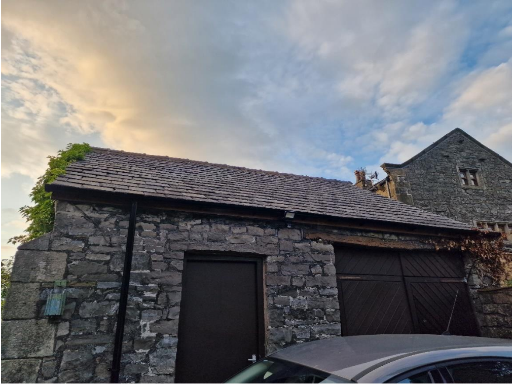
Photograph 3 – The southern aspect of B2
