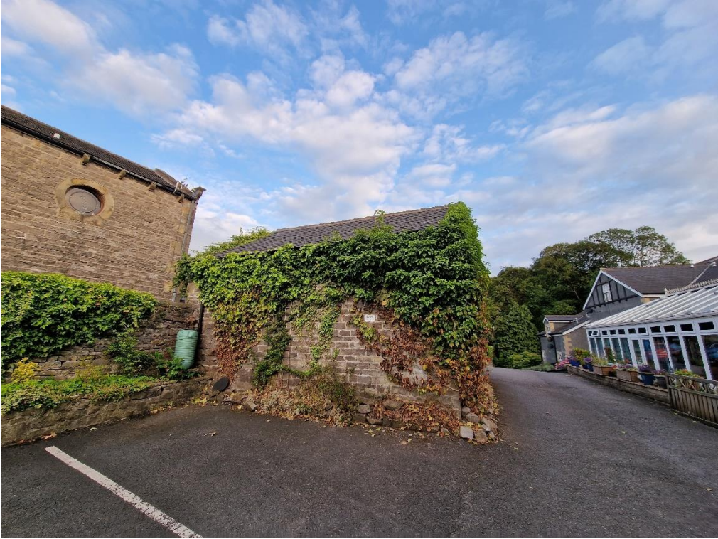
Photograph 1 – The northern aspect of B2
