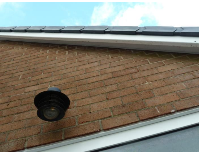
Photograph 4: General view of the dry verge and UPVC soffits with no means of bat ingress.
