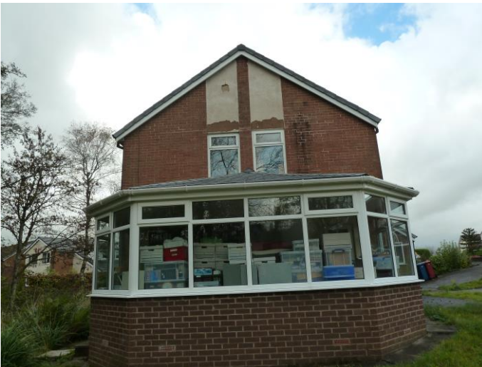
Photograph 3: South elevation – conservatory with composite slate roof. Blown render visible above.
