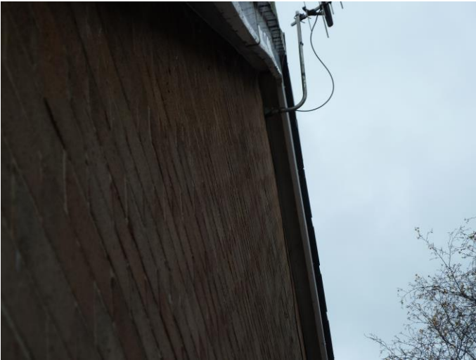
Photograph 2: Typical view of the tight-fitting UPVC soffits on the north gable. Dry verge visible.
