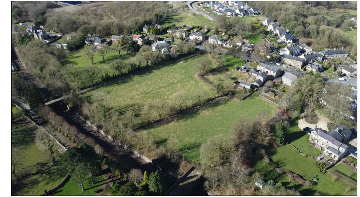
Aerial view of the site looking towards the southern & western boundaries
