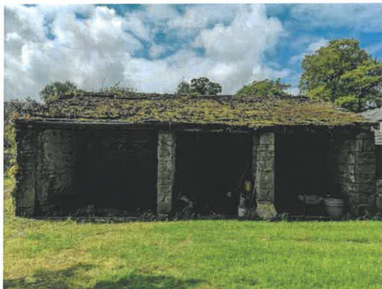
Figure 8.1.1: Open fronted stone garages
