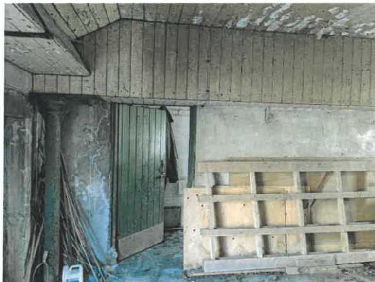
Figure 11.2.1: Internal view with ceilings present
