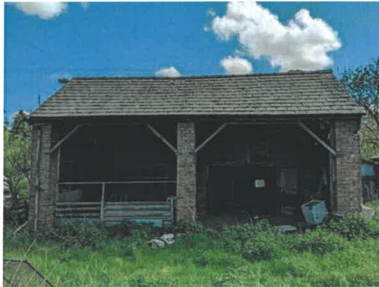
Figure 12.1.1: Open sided hay barn with brick piers and knee braced timber eaves structure
