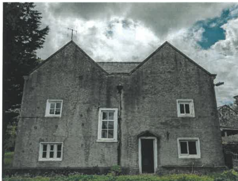
Figure 7.3.1: Front, north elevation. Twin northern wings, with central valley gutter and downpipe
