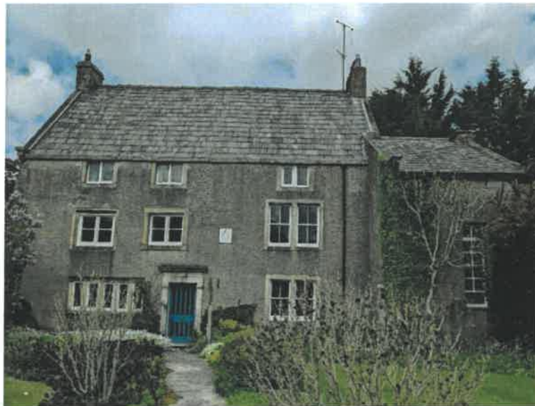
Figure 7.1.1: Rear, south elevation of the farmhouse and cheese press building
