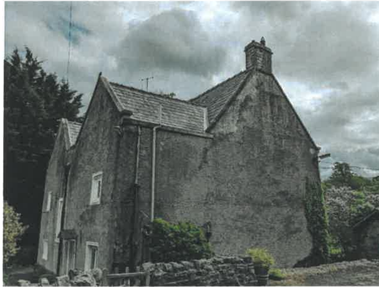
Figure 7.2.1: Side, west elevation. Northern wings to the left
