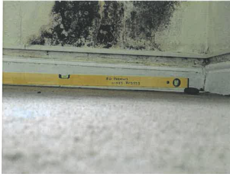
Figure 7.7.2: North east wing, floor dip to external corner
