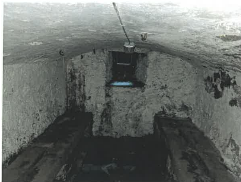
Figure 7.6.2: Basement cellar with stone arch ceiling
