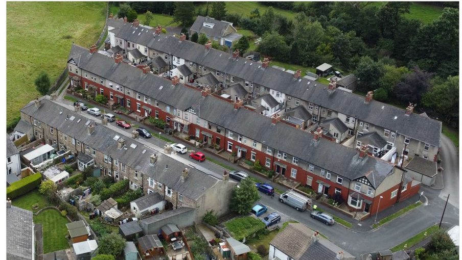
Stone, render and brick fronted terraced housing of Victoria Avenue
