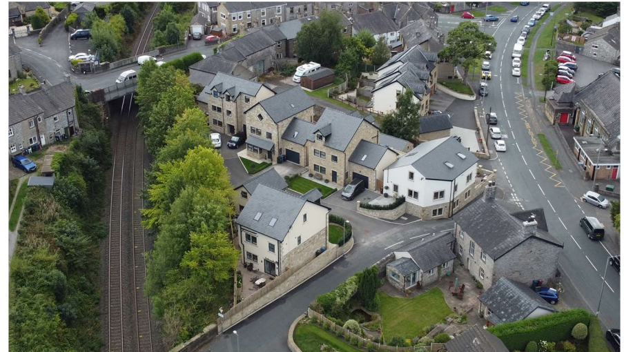
Recently built stone & render fronted mixed housing on The Cutting
