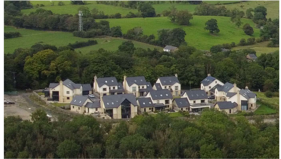
Recently built substantial family homes on Hare Hill Croft
