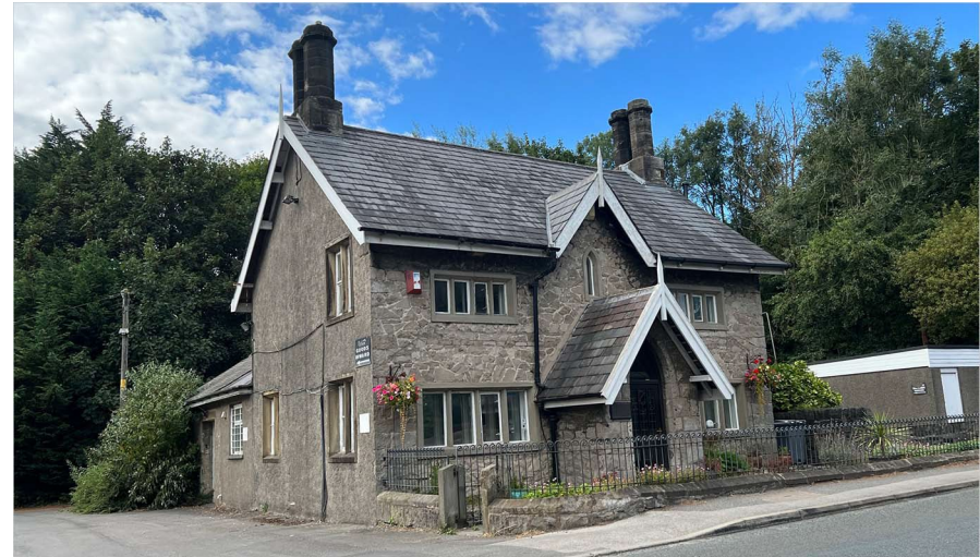
Stone built dwelling with gables & pikes
