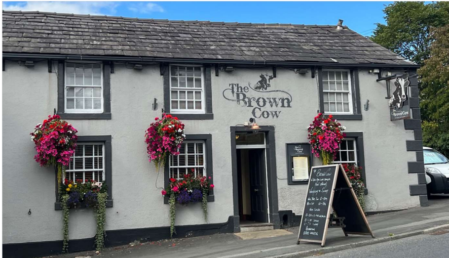
Rendered public house with simple facade
