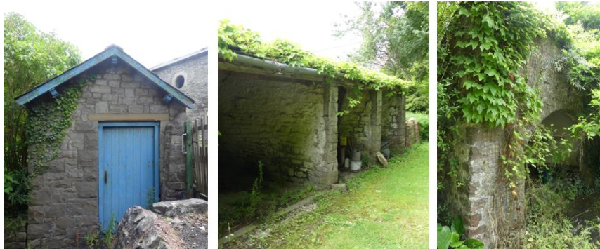
Figure 3.24: The store, garage and garden shelter incorporated into the perimeter of the garden
