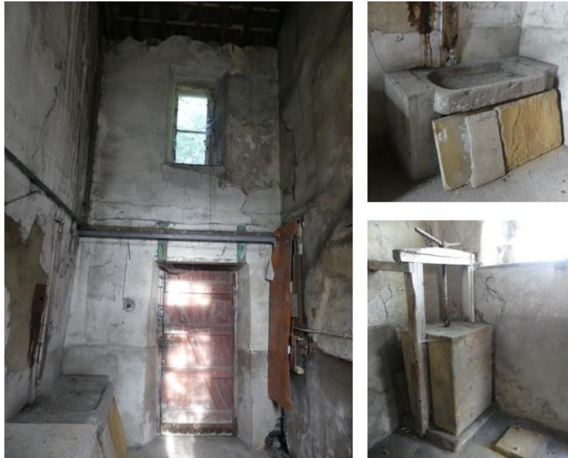
Figure 3.18: The interior of the double-height addition to the eastern gable
