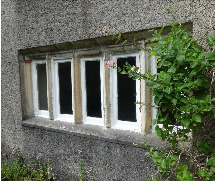
Figure 3.3: A five-light mullioned window remains to the left side of the door
