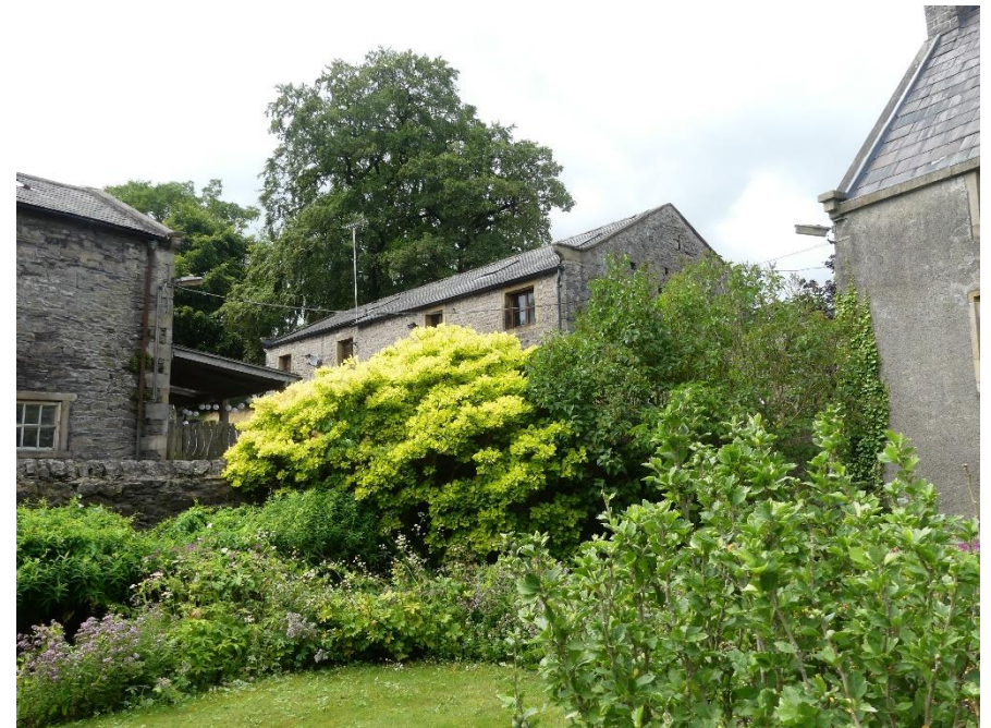
Figure 3.37: The rear (southern) elevation of the barn viewed between the house and dairy
