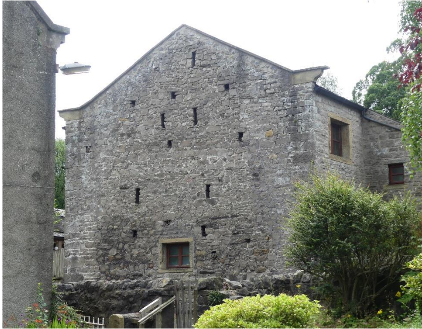
Figure 3.36: The eastern gable of the barn facing Crow Trees Farmhouse
