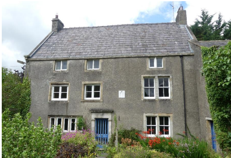
Figure 3.1: The southern elevation of Crow Trees Farmhouse
