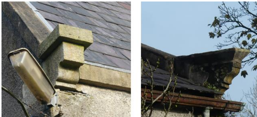
Figure 3.6: A kneeler to the main house (left) and the corresponding feature to the two-storey addition (right)
