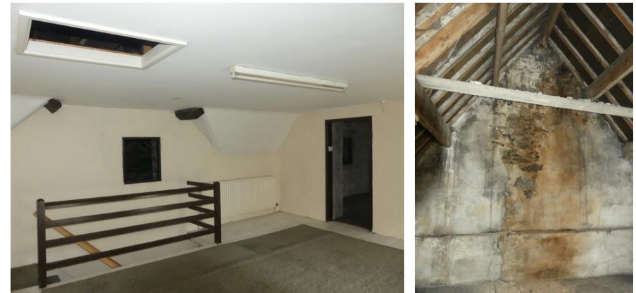
Figure 3.20: Damp penetration to the stairwell and north-eastern bedroom
