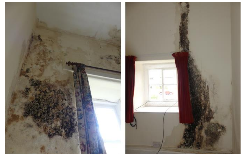
Figure 3.20: Damp penetration to the stairwell and north-eastern bedroom
