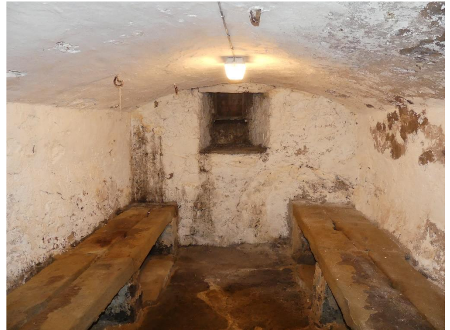
Figure 3.17: The cellar, below the eastern side of the main house
