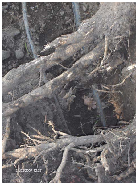
Typical root damage caused by excavation works
