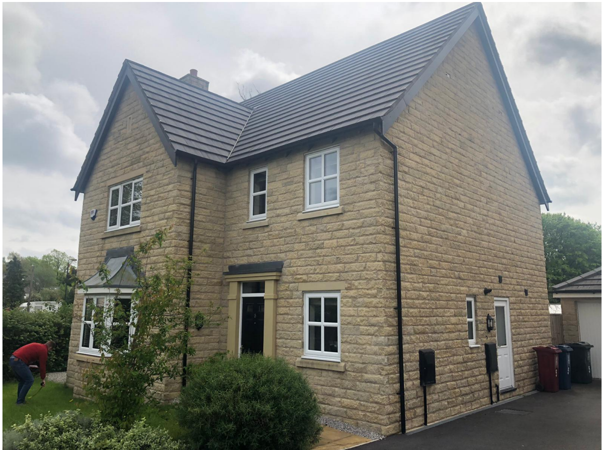
A view of the front (north) elevation and Gable (west) elevation.
