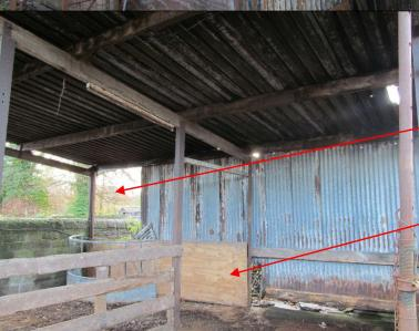
The internal space is extremely light, draughty and exposed due to the missing three sides and poor fitting roof
