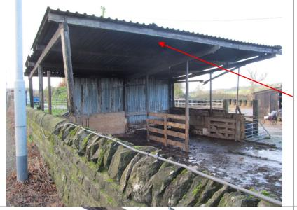
The structure is made from sheet metal panels over a steel frame with timber joists
