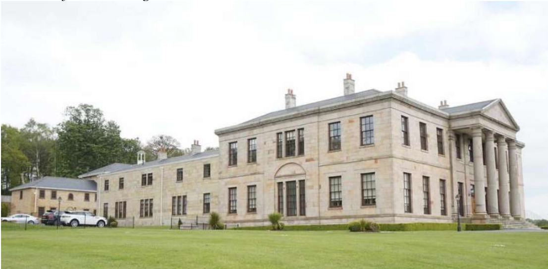
West elevation with similar tripartite window with blank segmental arch – a Samuel Wyatt favourite
