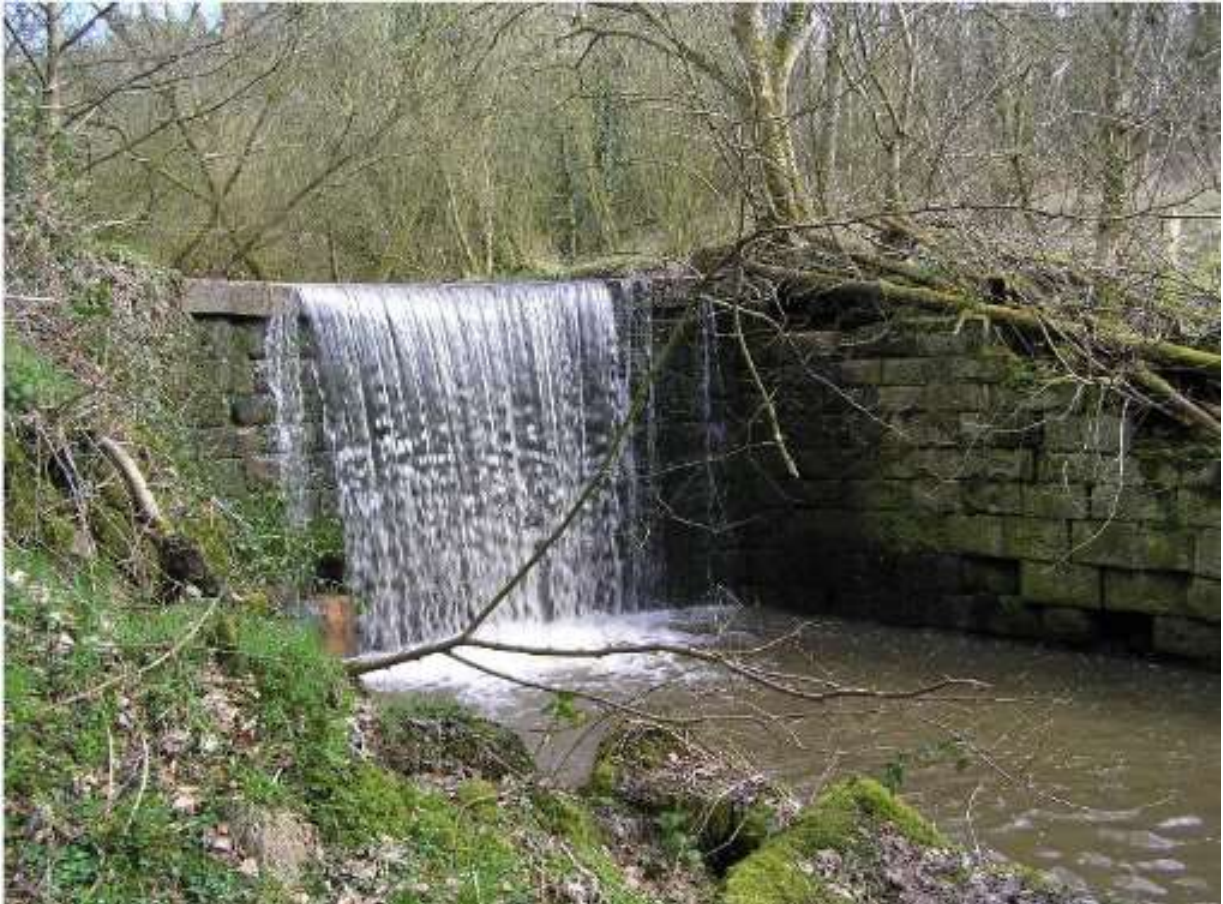
Typical weir on Arley Brook
