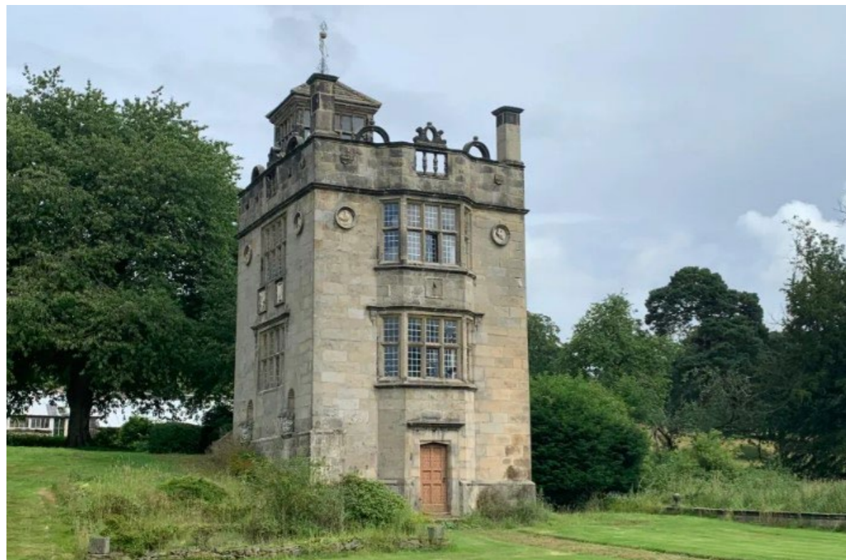
Otley Banqueting House
