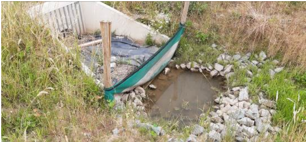
Silt fencing and straw bales installed across an inlet headwall within an attenuation basin, to promote settlement of silt within the concrete apron (where it can more easily be removed) prior to discharge into the attenuation basin. Coarse stone installed to dissipate flow and prevent scouring, and further promote settlement at the headwall
