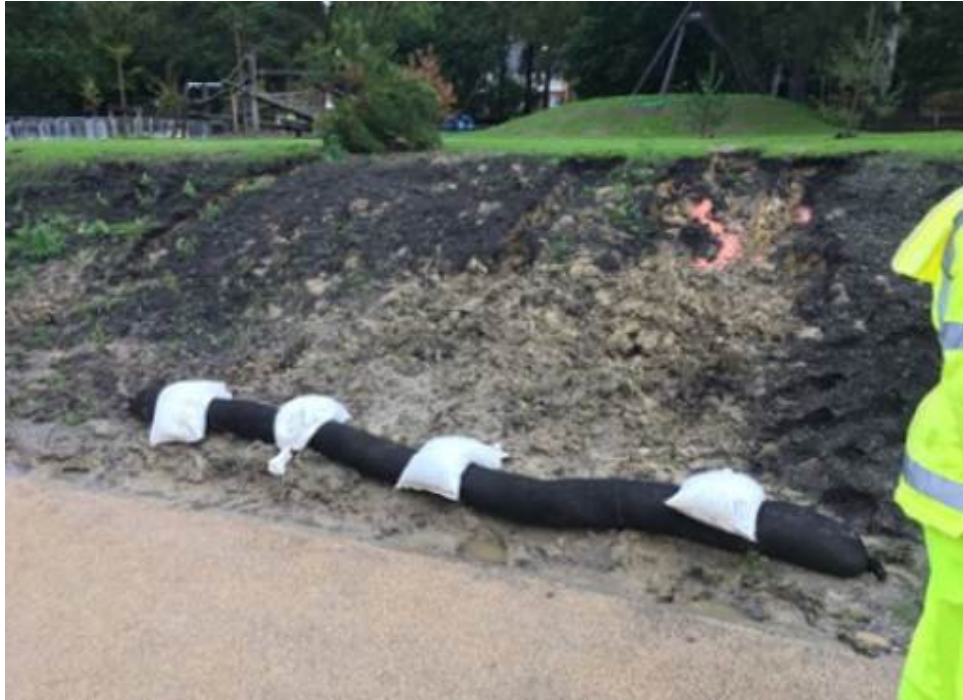
Silt Wattles utilised to intercept silt laden run-off from an unsurfaced slope (image courtesy of Frog Environmental)
