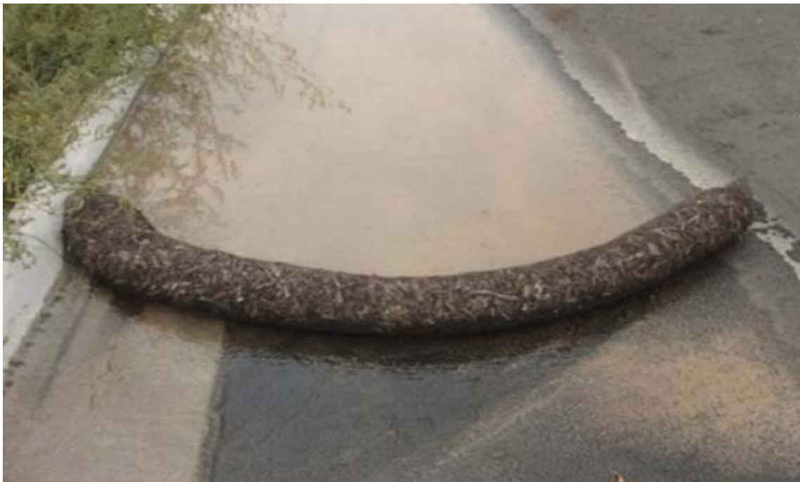
Silt Wattles utilised to intercept silt laden run-off on a road (image courtesy of Frog Environmental)
