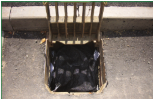
5. Close gully grid.
