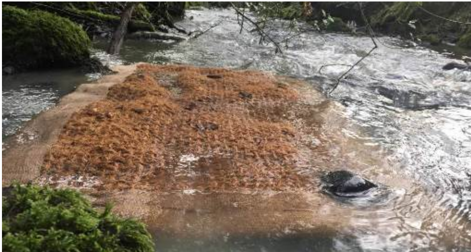
Placement of silt matting to capture settled silt downgradient within a surface watercourse (image courtesy of Frog Environmental)
