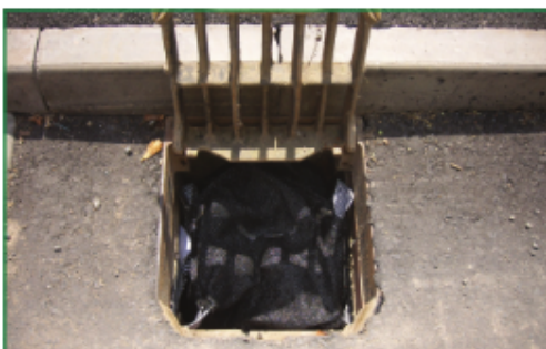
5. Close gully grid.
