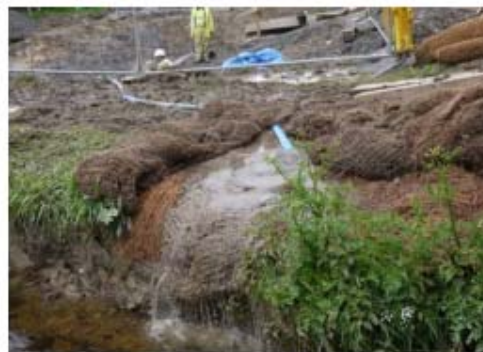
Deployed to treat muddy excavation water
