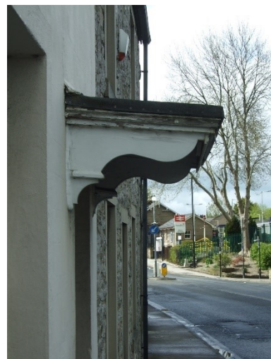
Picture 9 - Timber hood to #13
