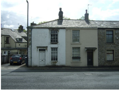
Picture 4 – West elevation along Railway View Road
