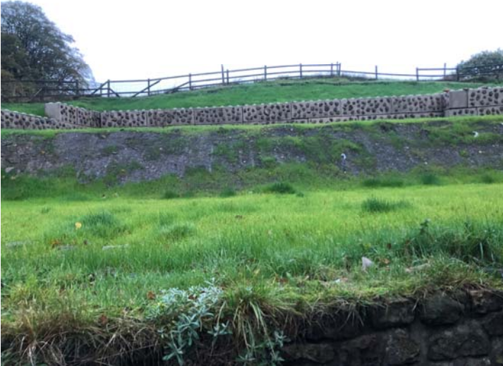
'Gorilla' blocks in place indicating more level terraced lawns.
