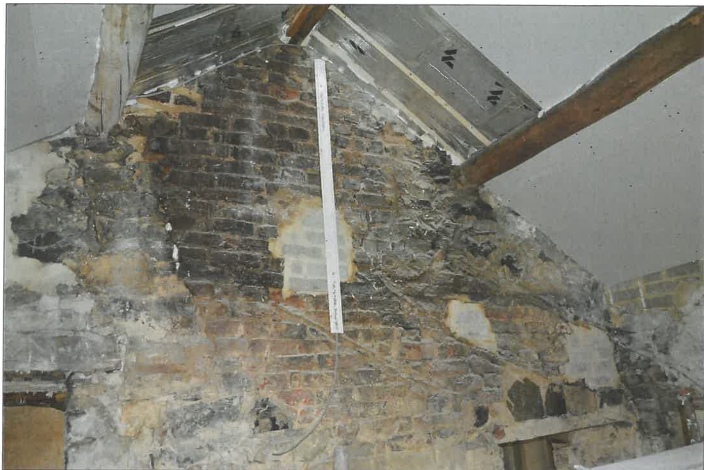
PL48: View of brickwork flues to the west wall of the first floor south east unit.
