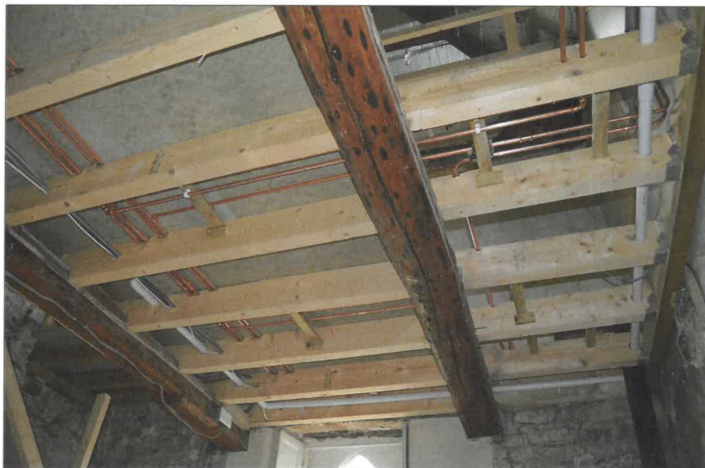
PL27: View of modern floor structure installed over former ground floor kitchen.
