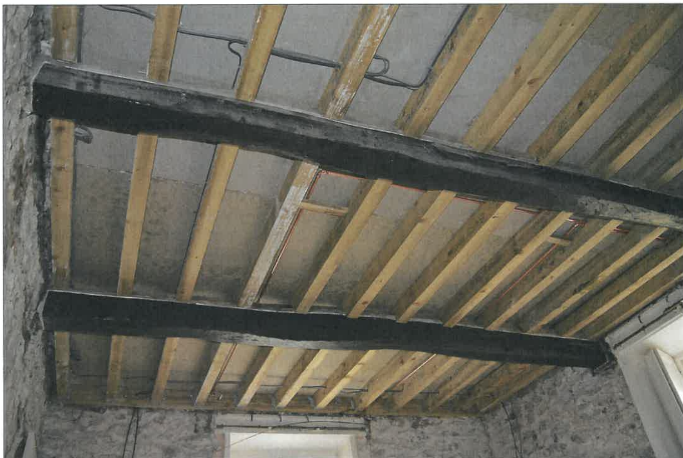
PL32: View of the modern floor structure installed over the ground floor south east unit.
