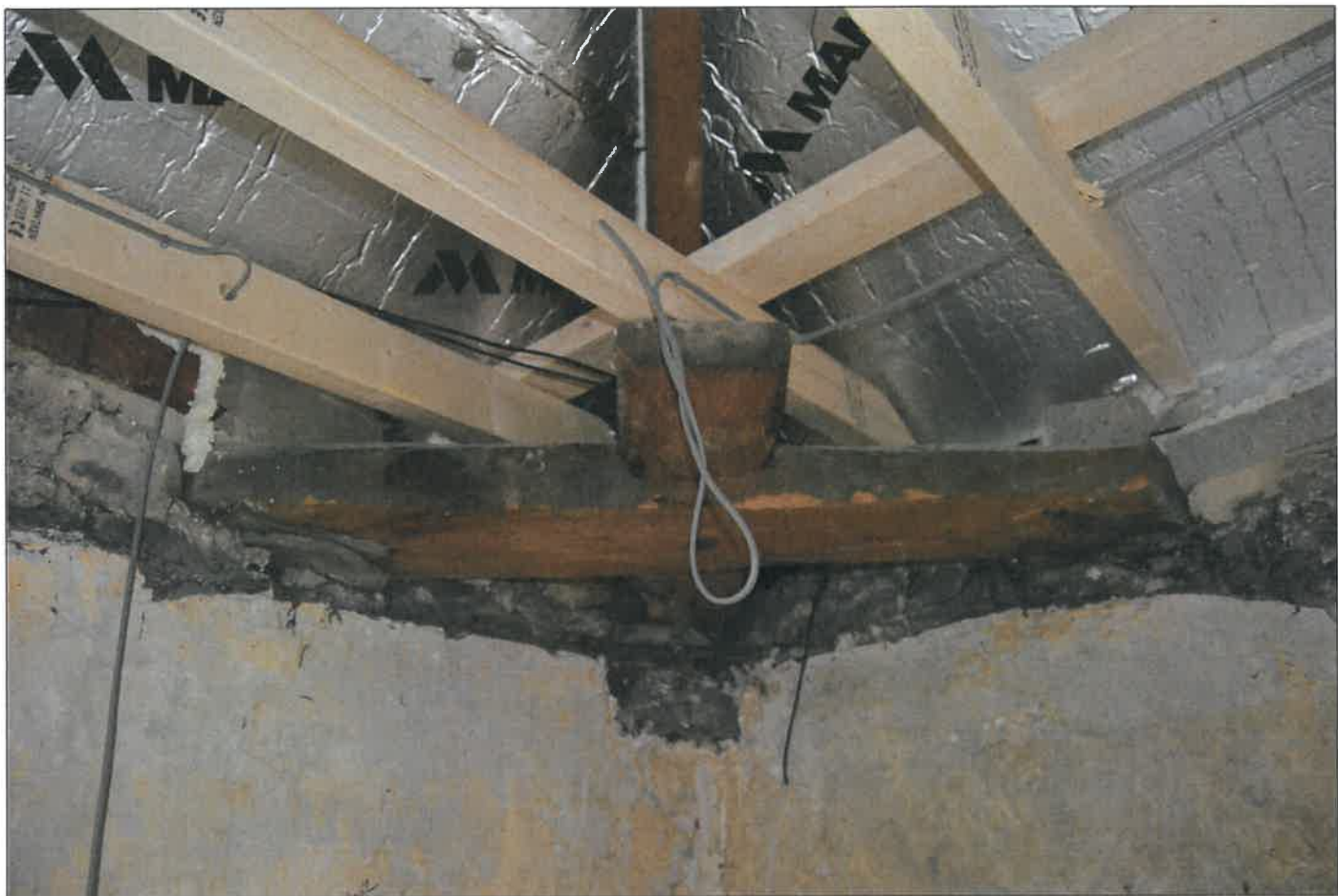
PL41: View of exposed timber dragon tie to the south west corner of the first floor south west unit.
