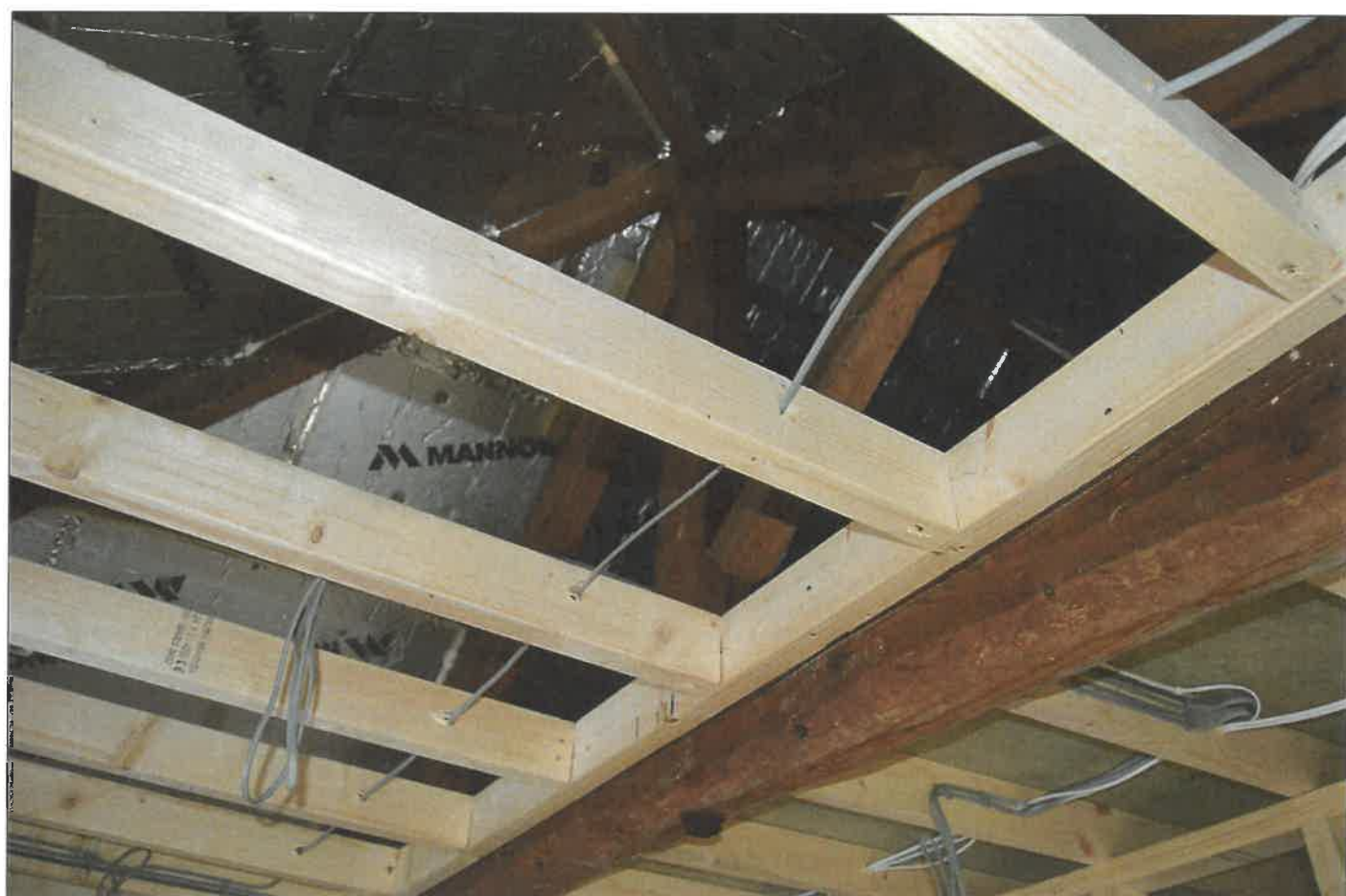
PL40: View of timber king post roof truss over the first floor south west unit.
