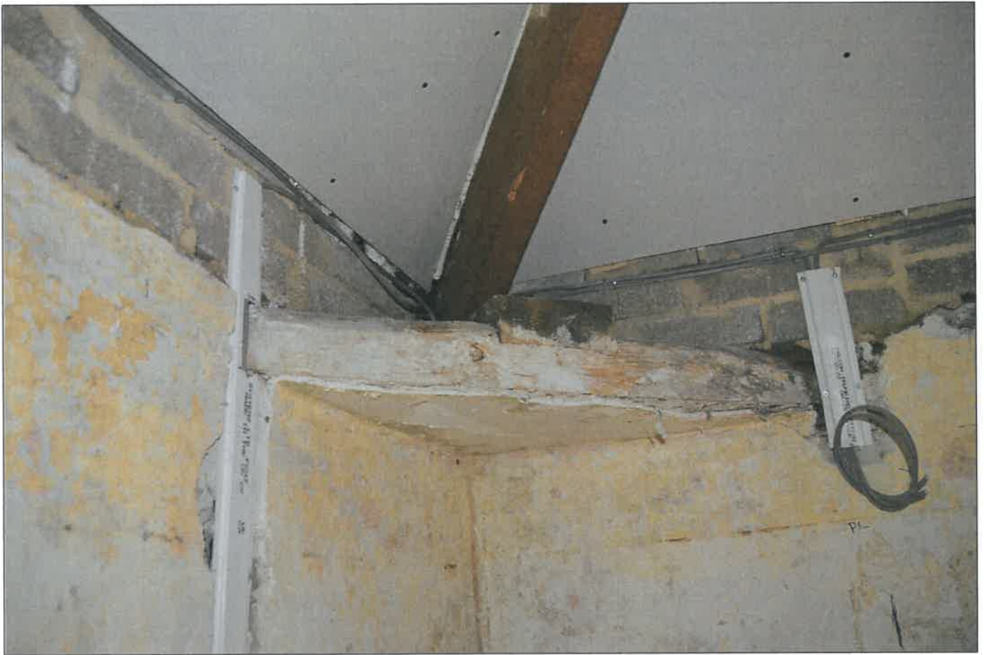
PL50: View of the dragon tie to the north east corner of the first floor south east unit.
