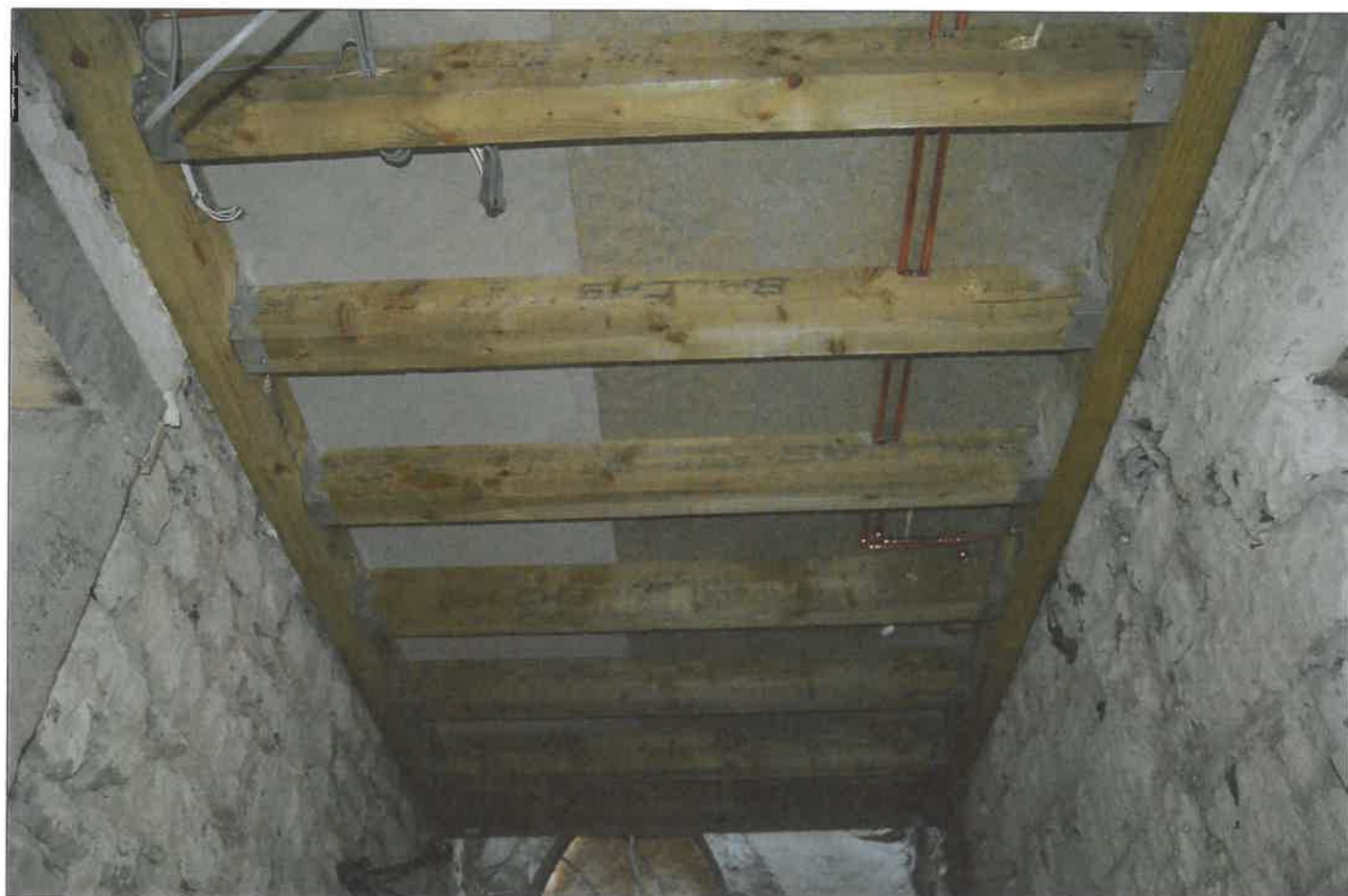
PL18: View of modern floor structure installed over the ground floor inner hallway.
