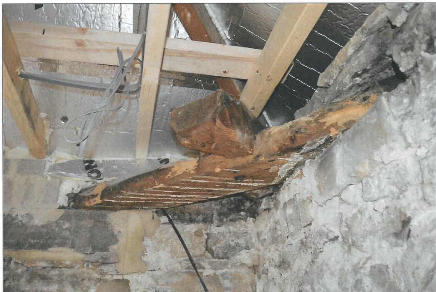
PL42: View of exposed dragon tie to the south east corner of the first floor south west unit.
