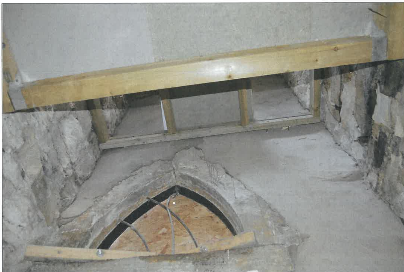
PL16: View of void formed to first floor structure adjacent external door to ground floor inner hallway.
