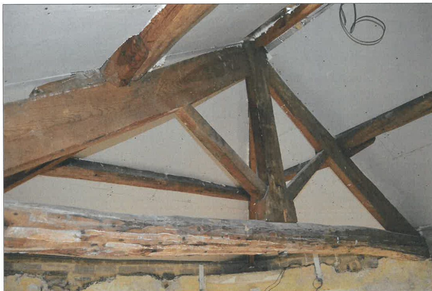
PL46: View of timber king post roof truss to the first floor south east unit.
