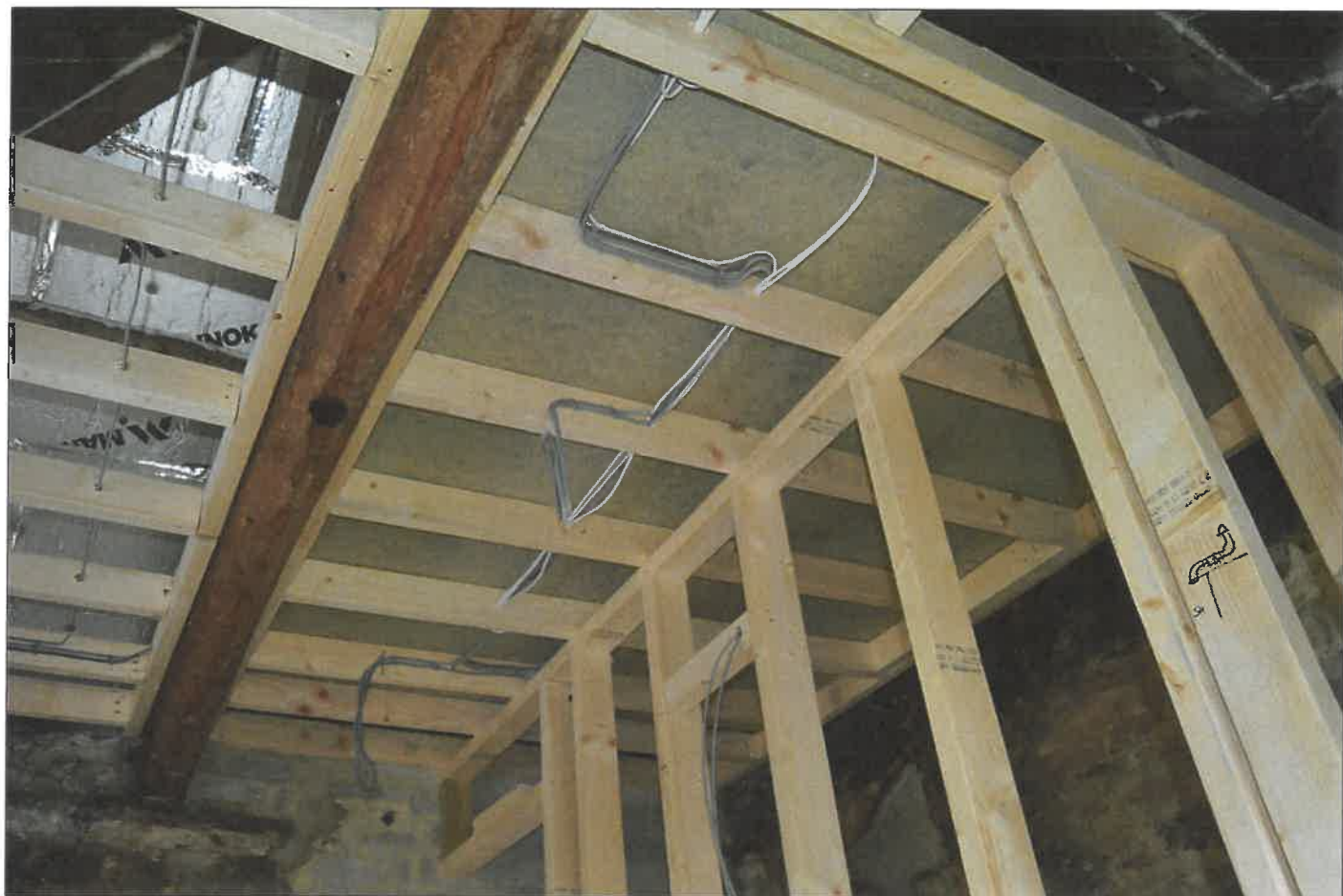
PL39 View of modern ceiling structure over first floor south west unit and staircase.
