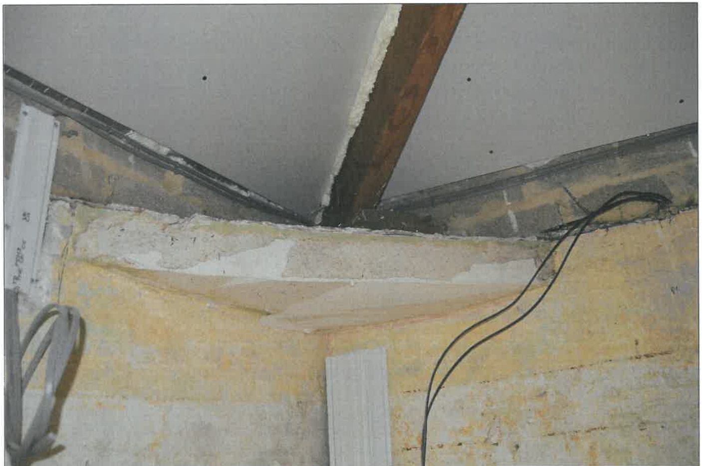
PL51: View of the dragon ties to the south east corner of the first floor south east unit.
