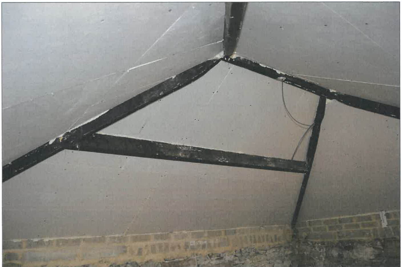
PL59: View of the plasterboard ceiling lining to the first-floor north unit.
