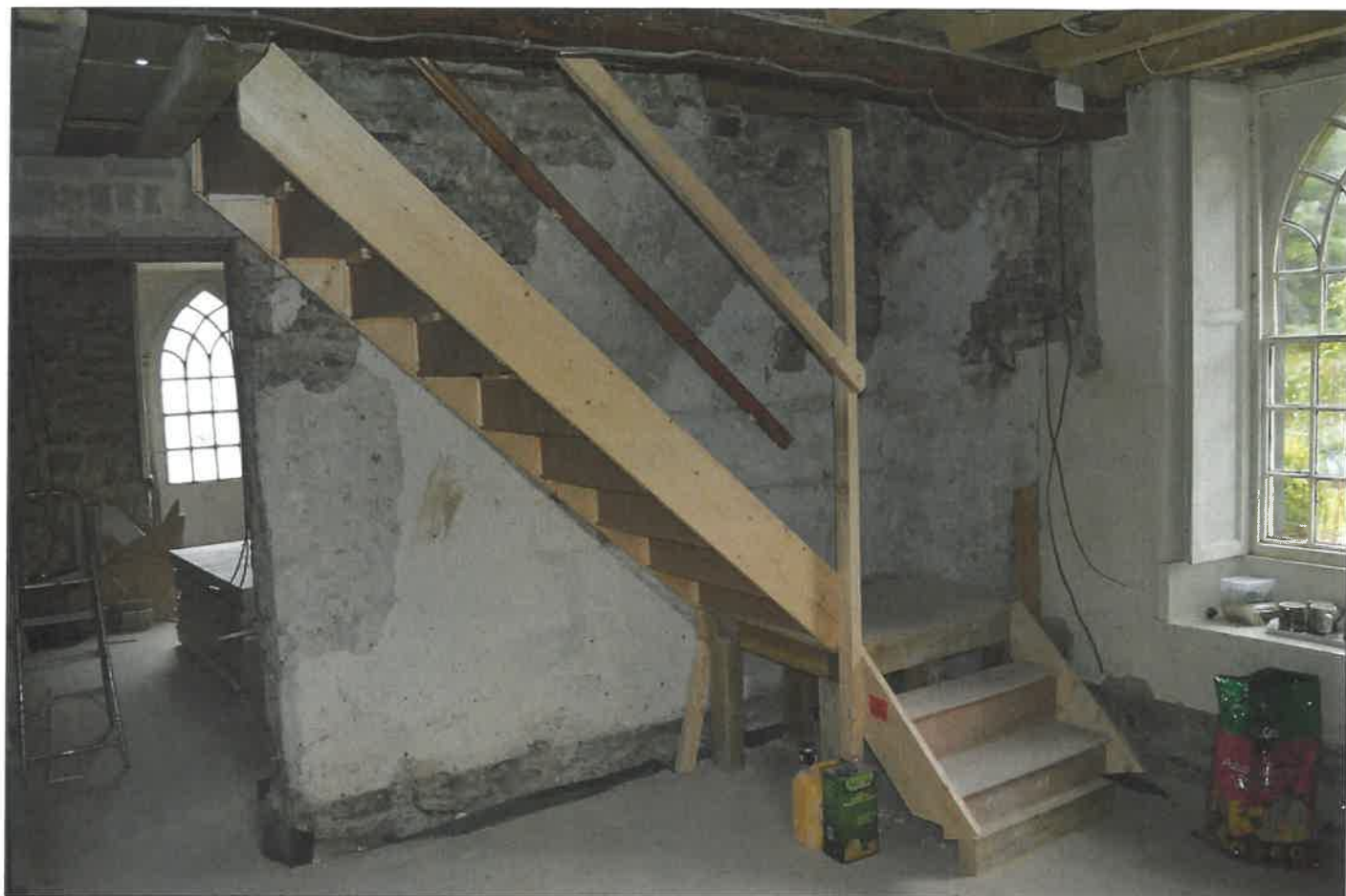
PL26: View east within former ground floor kitchen showing temporary staircase following the removal of the former staircase.
