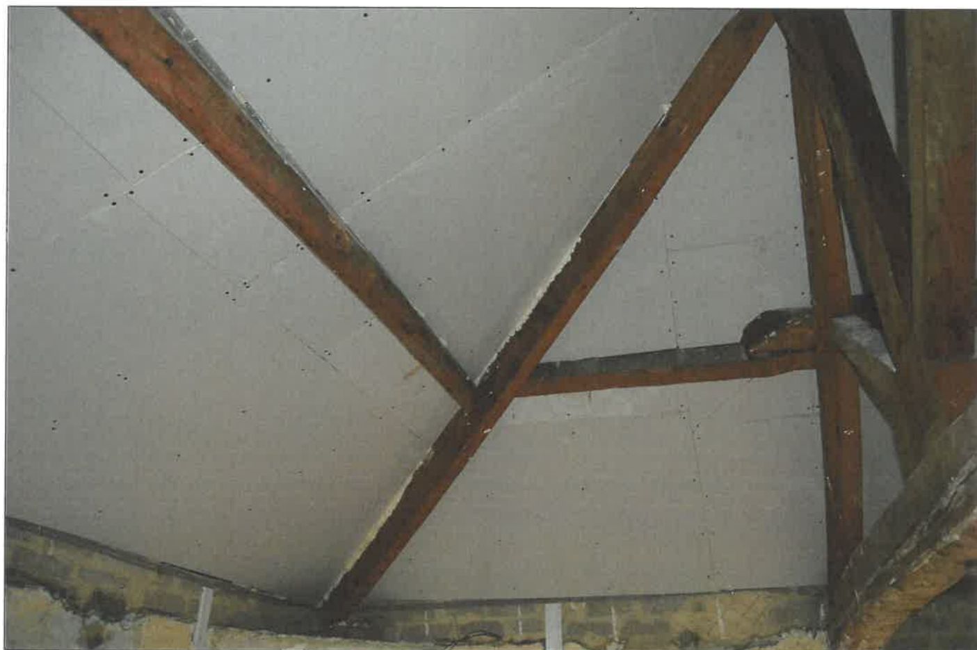
PL49: View of plasterboard ceiling linings to the first floor south east unit.
