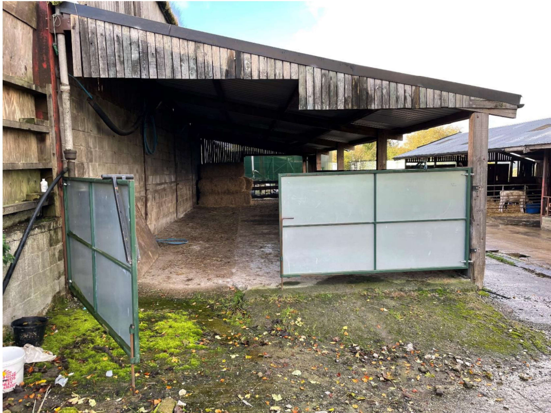
Building to remove
