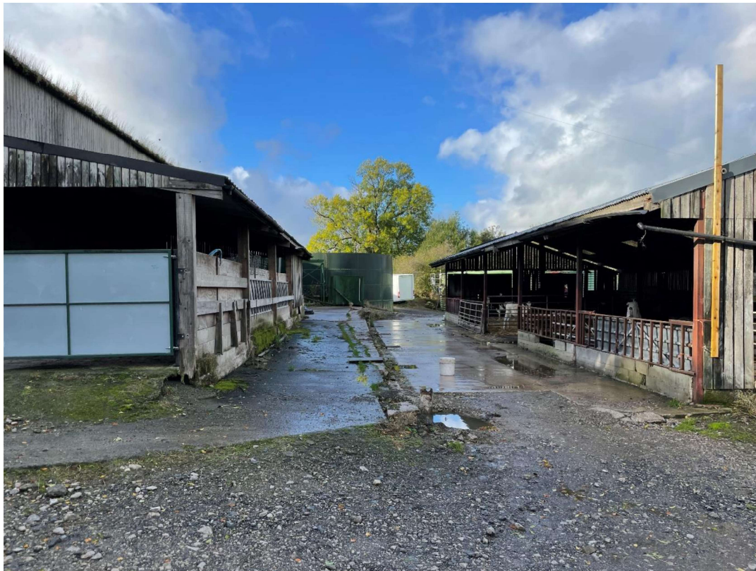
Open yard area to cover
