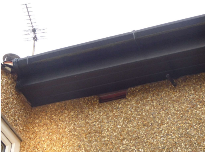
Rear elevation well sealed soffits no gaps.
