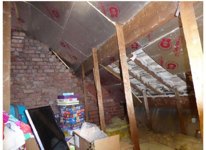
Loft space with partial insulation board under slates.
