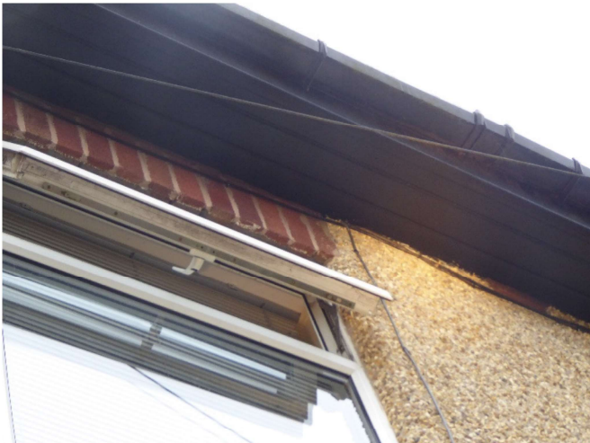
Front elevation well sealed soffits no gaps.
