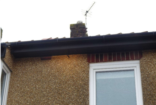
Rear elevation well sealed soffits no gaps.
