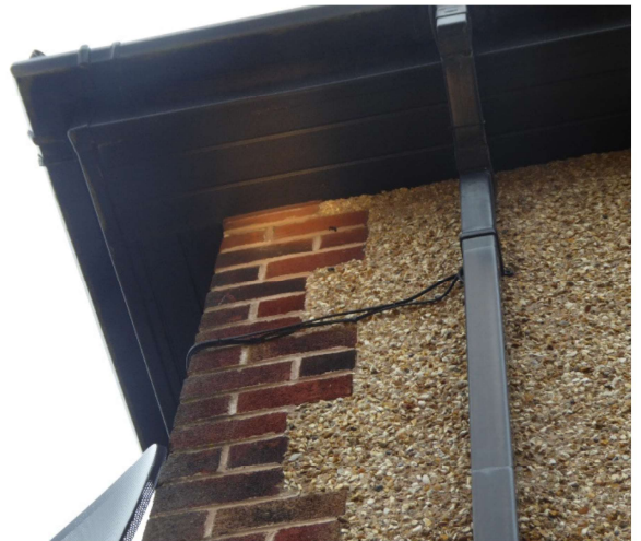
Front / corner side elevation well sealed soffits no gaps.
