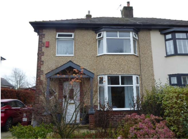
Front elevation general view. No slate / roof gaps / points of potential ingress.
