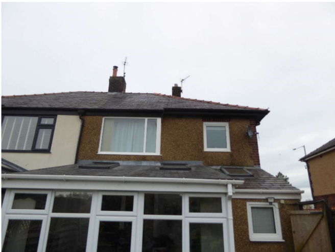
Rear elevation well sealed soffits no gaps. No slate / roof gaps or points of potential ingress.
