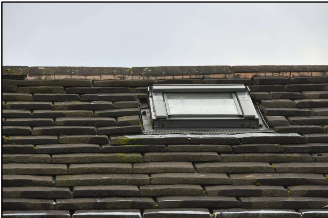
View of roof coverings with Velux windows
