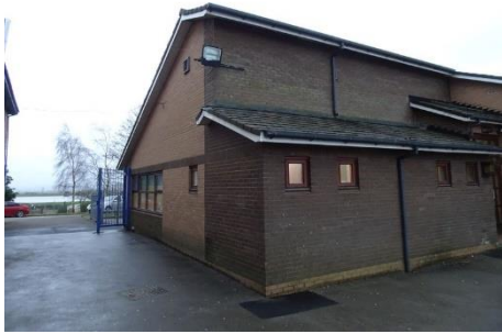
East and north facing elevations
