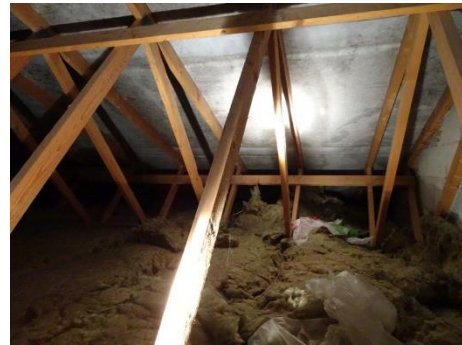
Inside loft facing north
