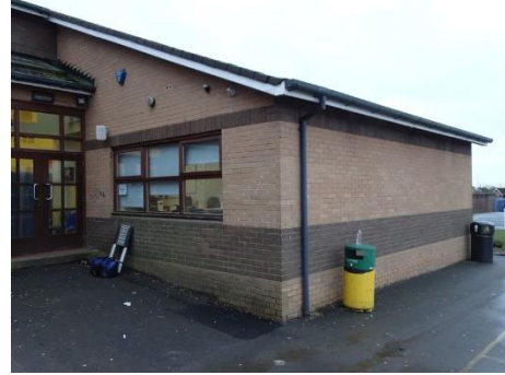
North facing entrance and north facing elevation
