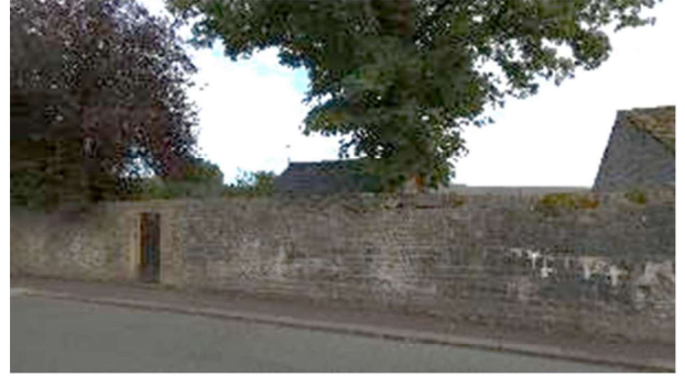
PLATE 2: Looking south across Downham Road towards the Site boundary, towards the stone shed (B1)
