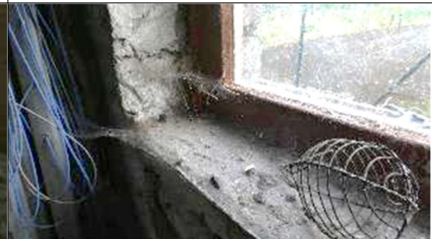
PLATE 14: Building B1, south facing windowsill.
