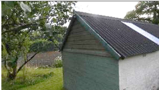
PLATE 19: South-eastern aspect of the gable end. Brick built gable end with tight fitting tongue & groove cladding
