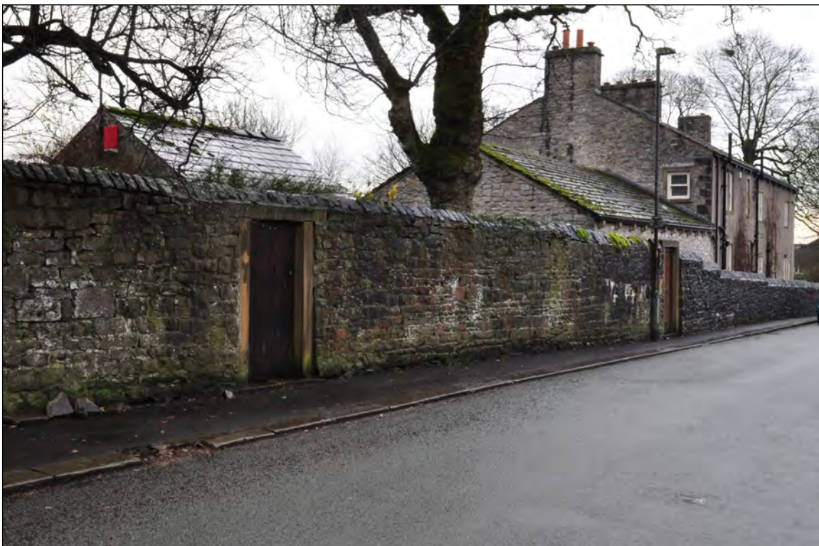
Photo 2: Boundary wall on Downham Road.
