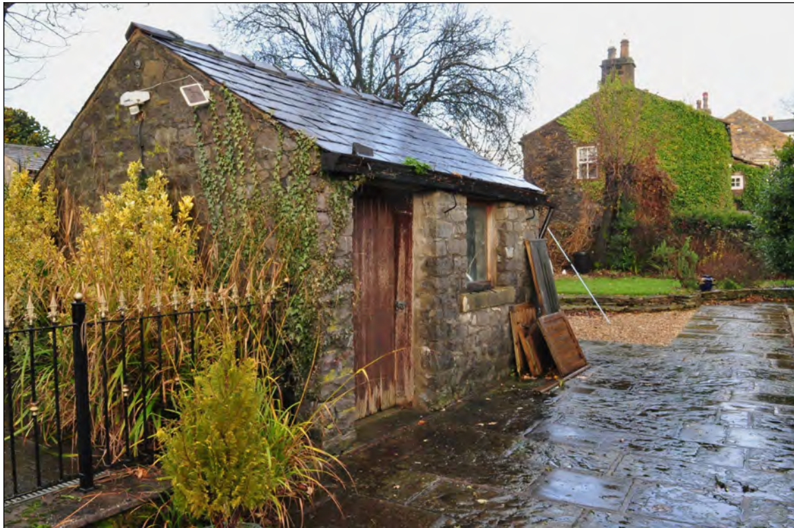
Photo 7: Outbuilding proposed for demolition.
