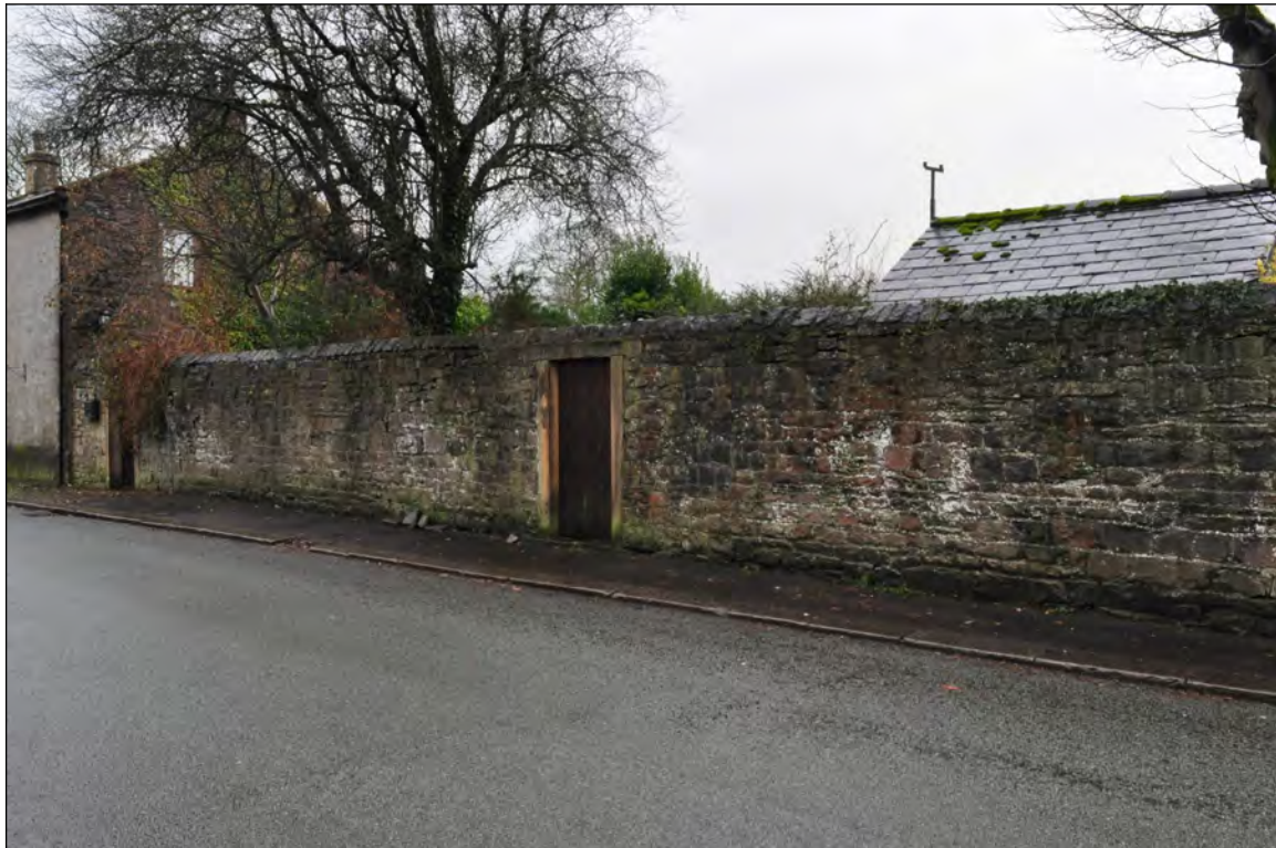
Photo 3: Boundary wall on Downham Road, number 53 at left.
