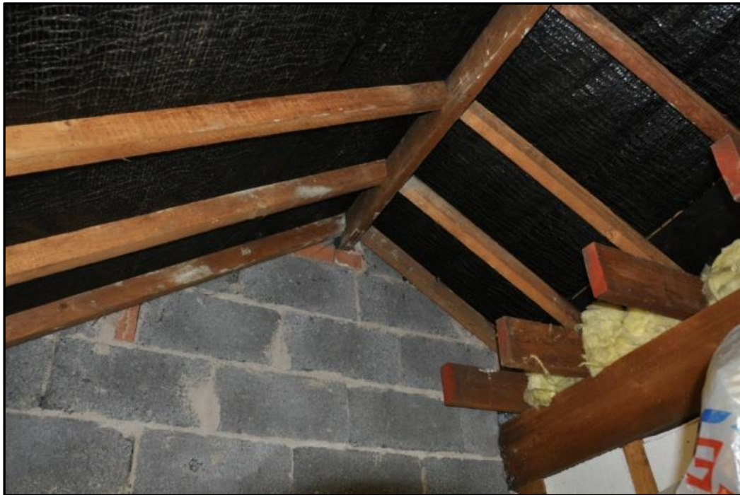
Image showing roof void with intact liner, mortared block walls and rock wool
