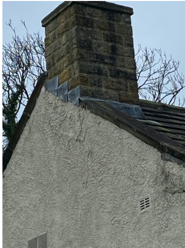
Photograph 4: Gable elevation at chimney breast viewed from rear bedroom
