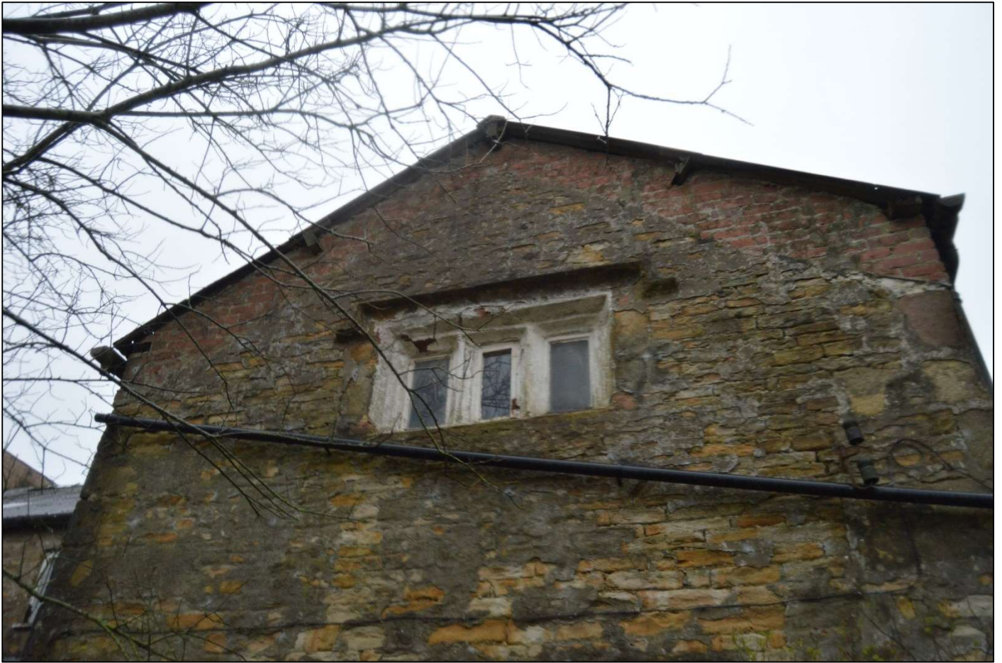
PL07: View of the three-light, stone mullioned window to the first floor of the cross wing.
