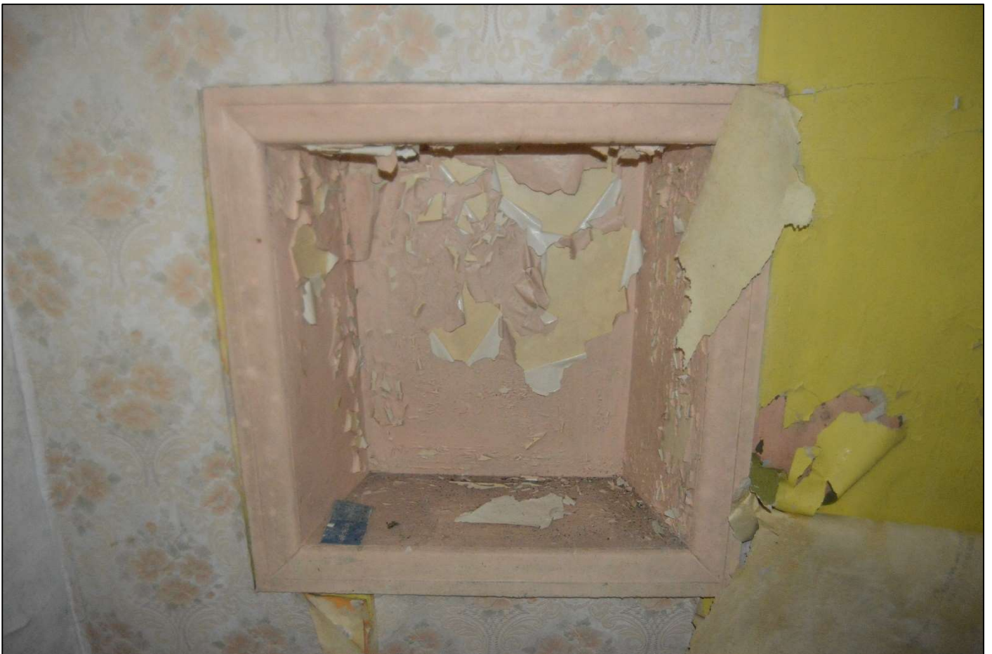
PL36: View of blocked possible former staircase window to the first-floor landing to the rear of the cross wing.
