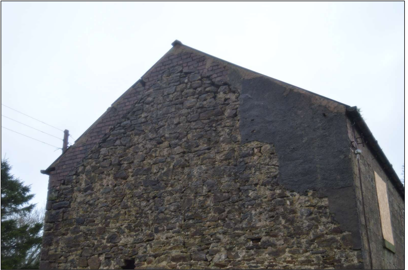
PL17: View of raised roof and old roofline to the west gable end elevation.
