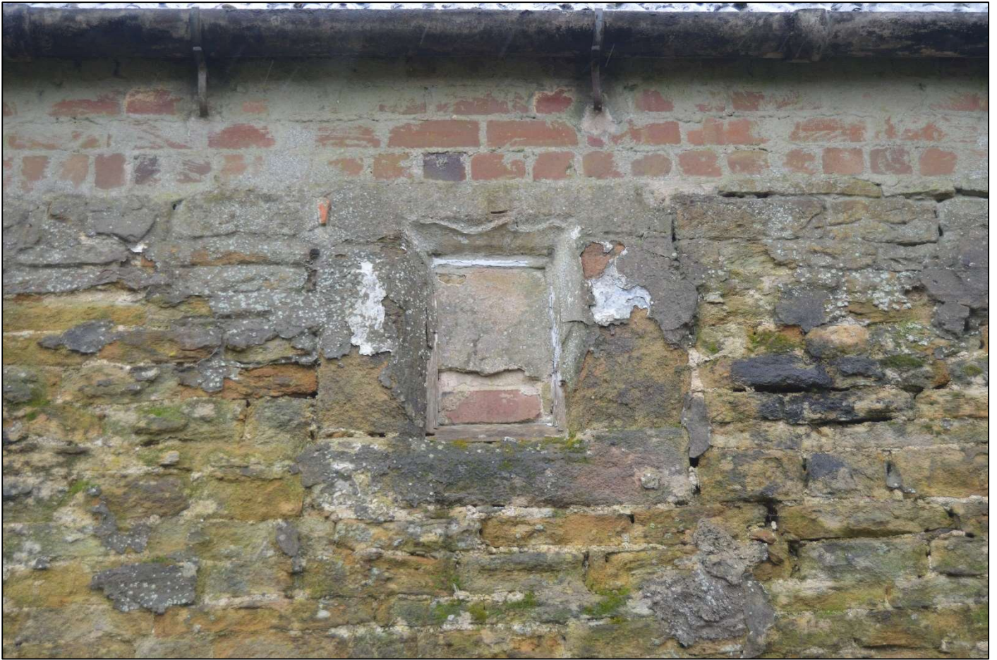
PLI 5: View of blocked up former staircase window to the first floor of the rear north elevation.
