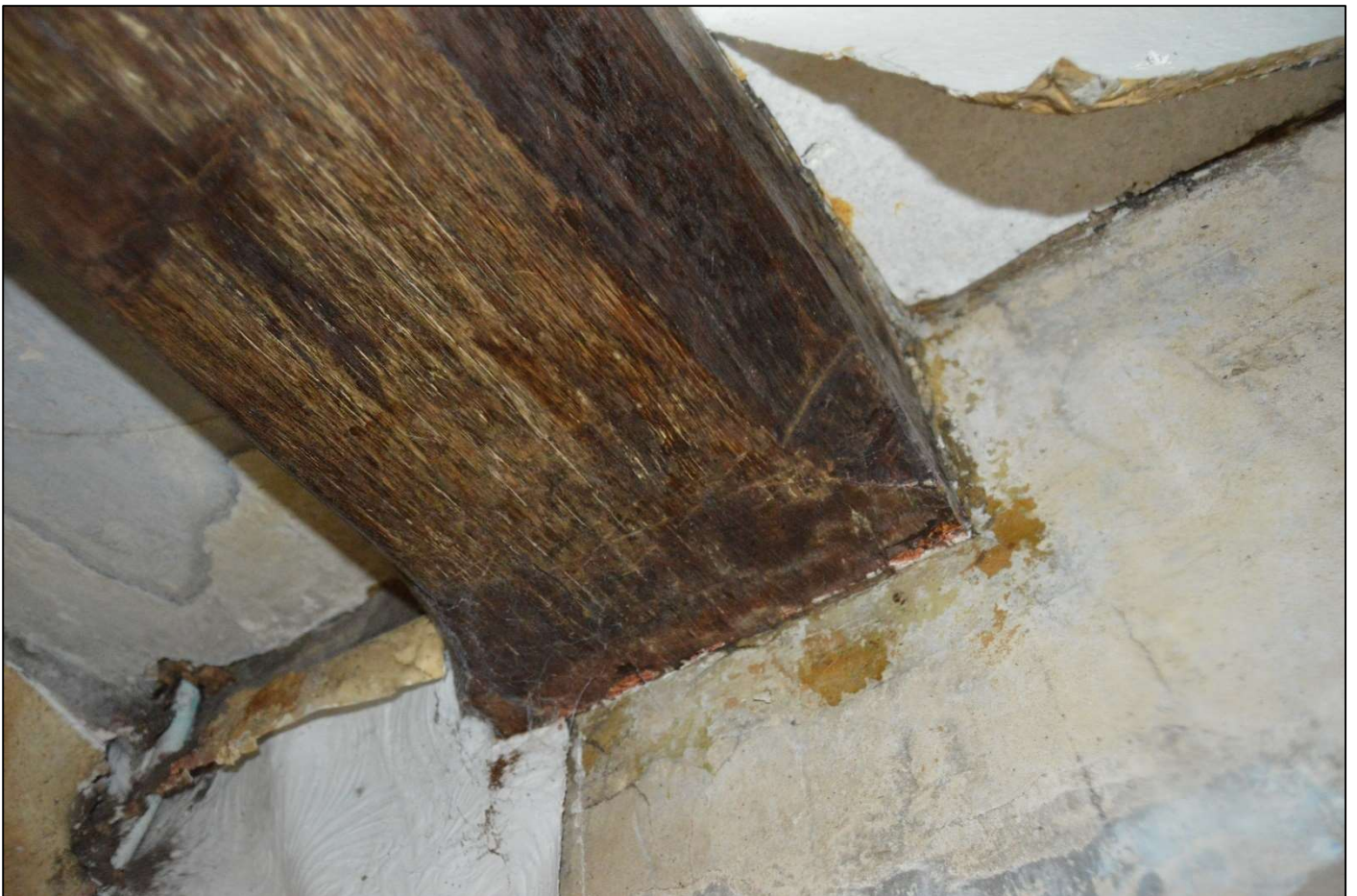
PL31: View of 17 th century floor beam within the central ground floor unit, with chamfers and stops.
