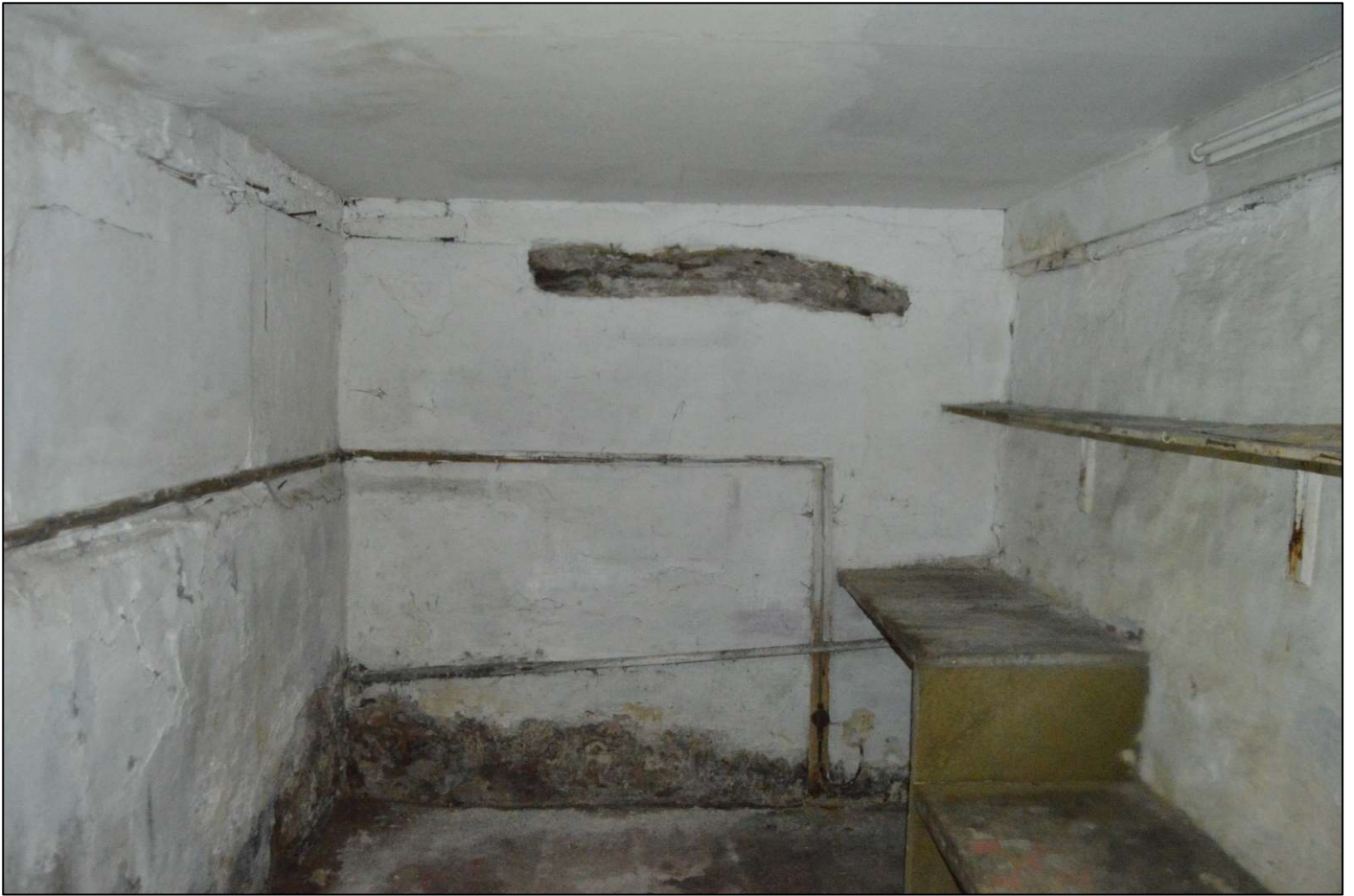
PL26: View east within the rear ground floor unit to the cross wing (note the timber lintel to the blocked window).
