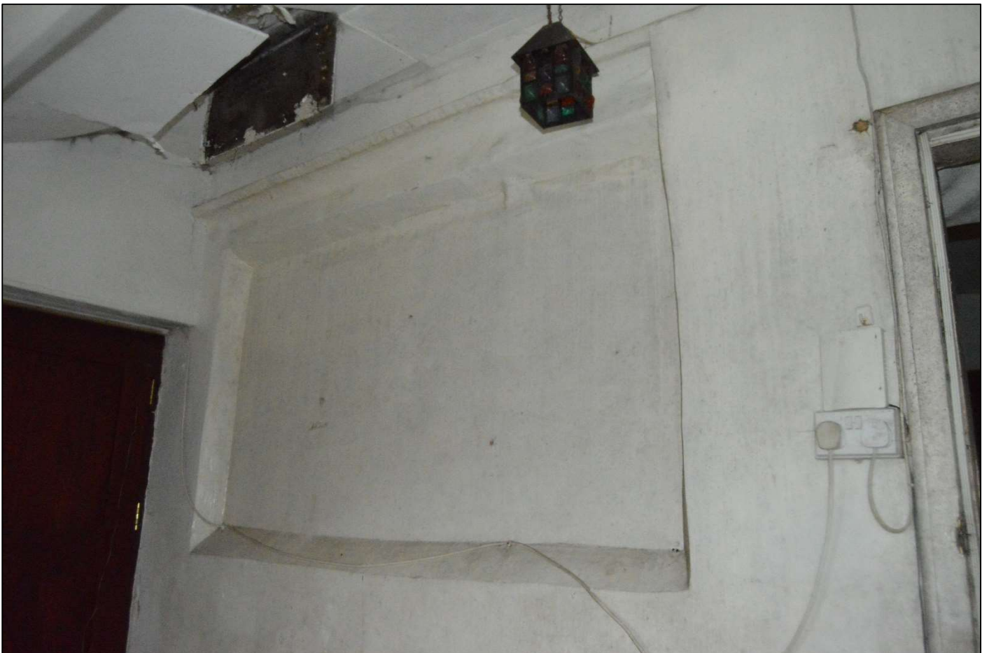
PL25: View of blocked former mullioned window from within the front south elevation lean-to.
