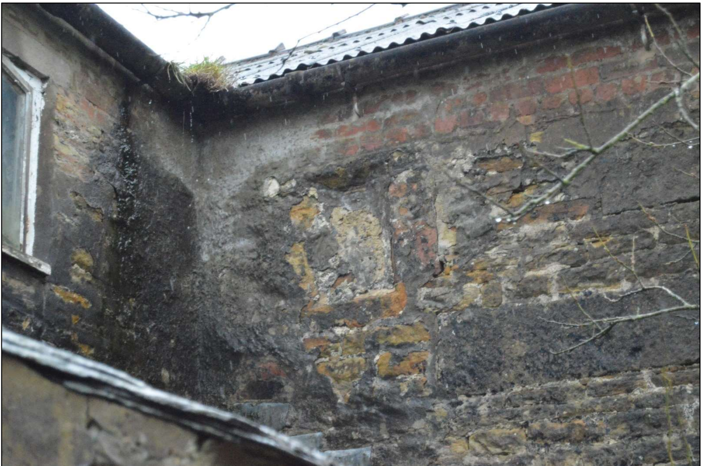
PL04: View of blocked window to the first floor of the west elevation of the cross wing.
