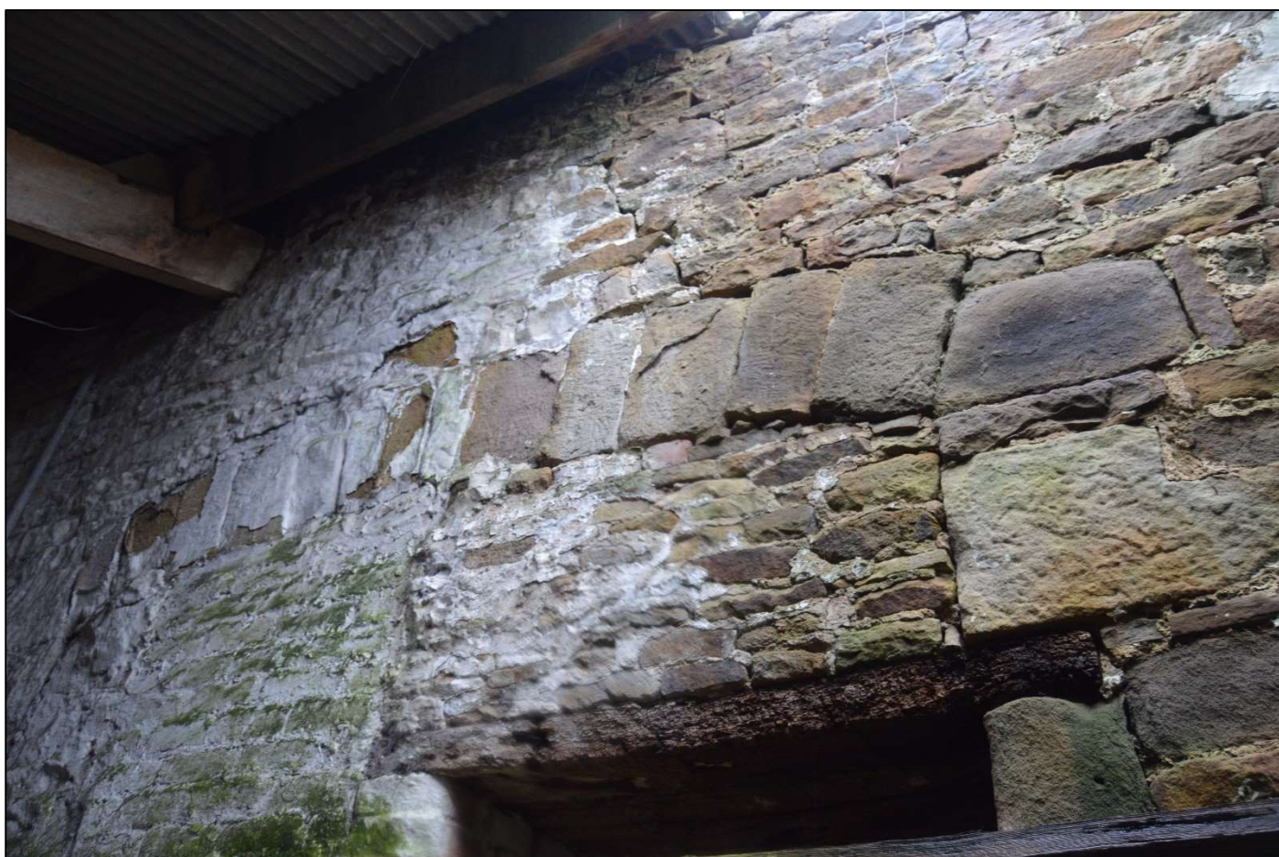
PL62: View of stone voussoirs to the blocked-up opening viewed from within the south shippon.
