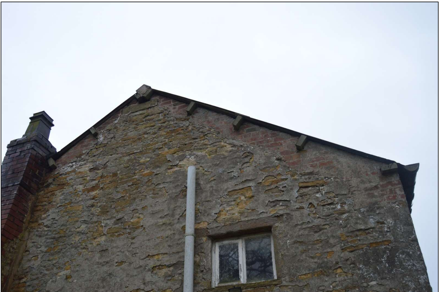
PL10: View of raised roof and old roofline to the east gable end.
