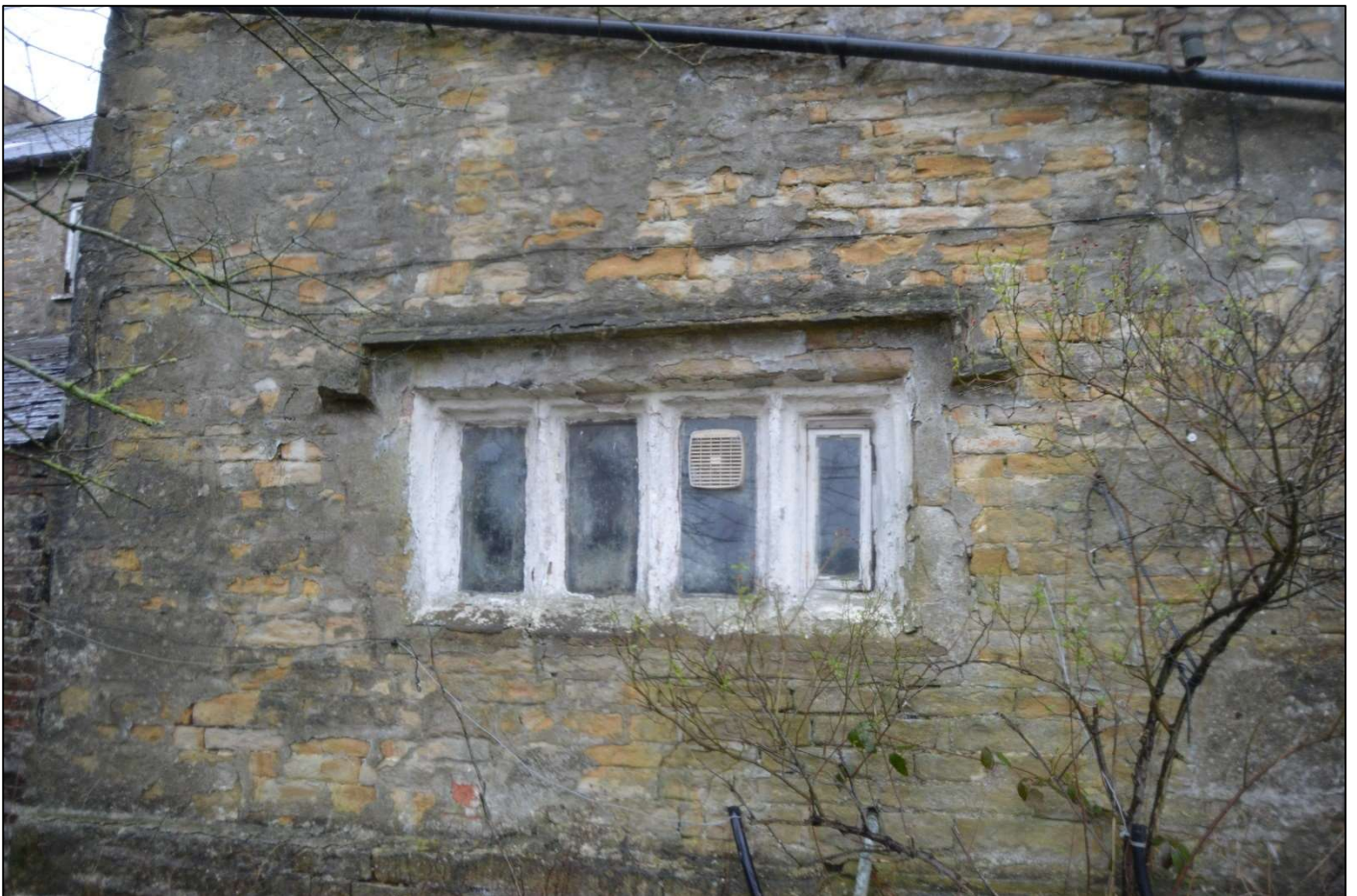
PL06: View of the four-light, stone mullioned window to the ground floor of the cross wing.
