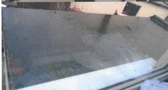
Flat roof from above.
