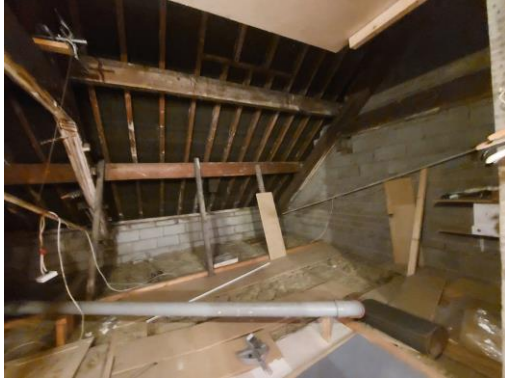
Plate 4: View of loft void, fir wall and low wall along lower roof section.
