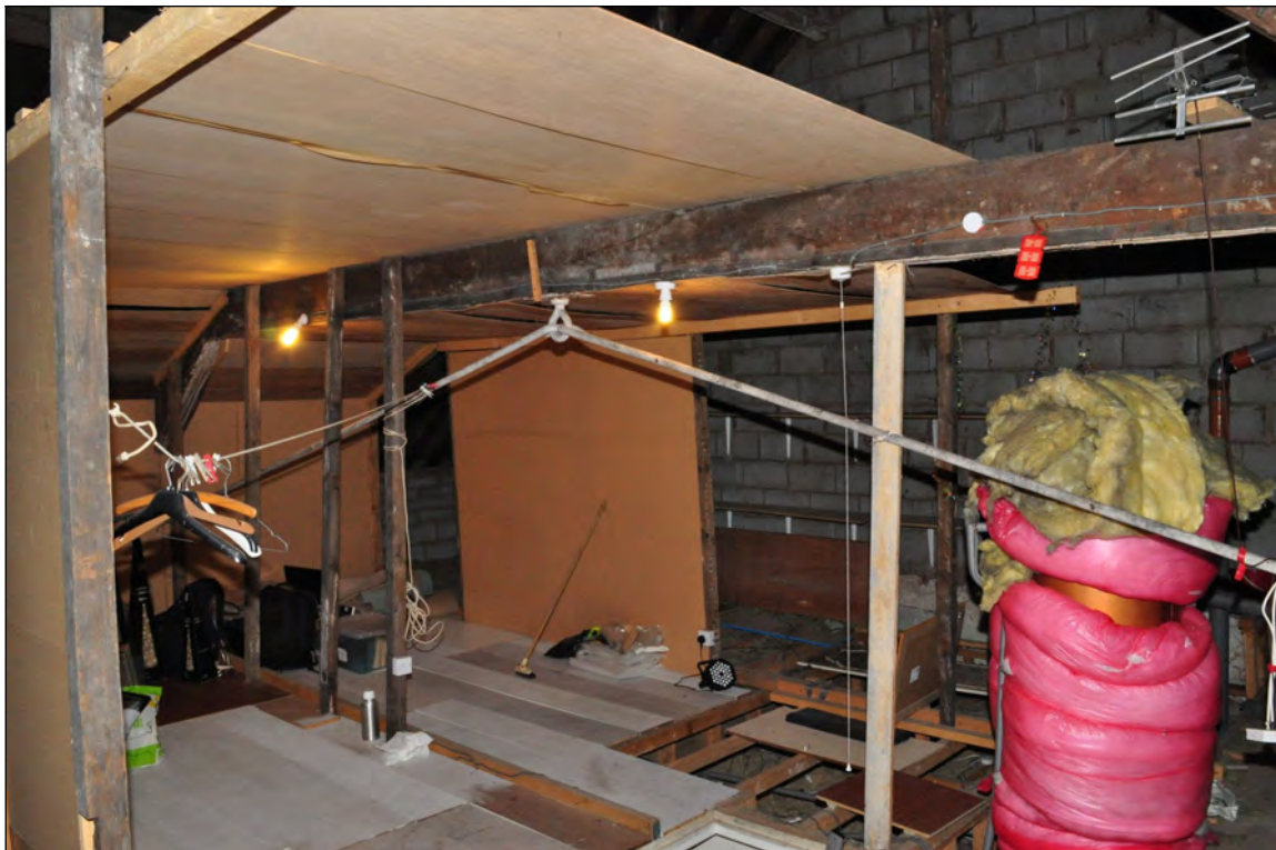
Photo 3: Roof space over Flat 3. Upper storey originally extended up to the collar, which retains traces of lath and plaster.
