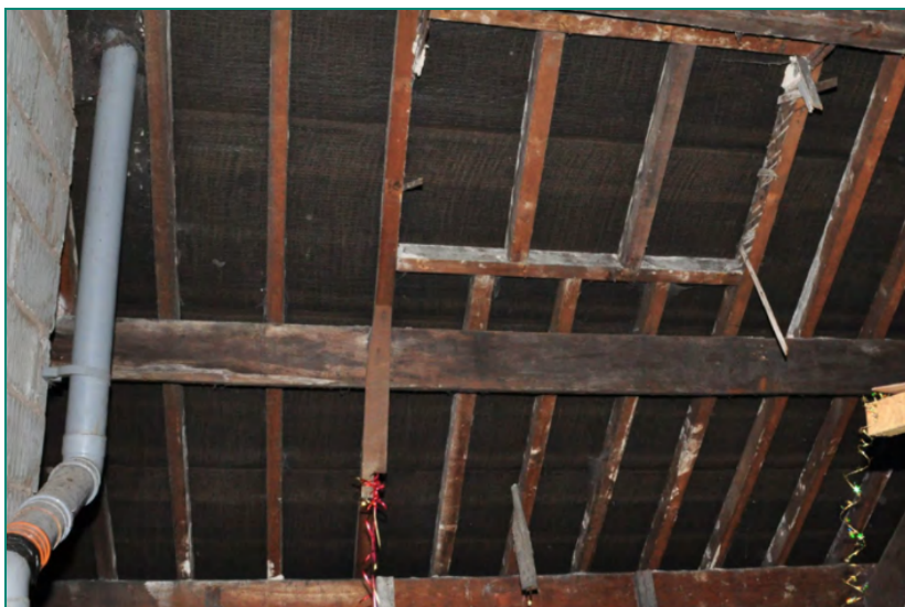
Photo 4: One of two former rooflights in west side, with remnants of lath and plaster lightwell to sides
