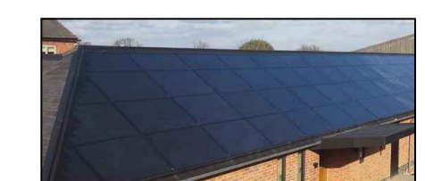
Proposed south-west facing roof to be finished with GB SOL Seamless Infinity Solar Roof system
