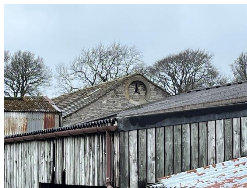
Photograph 2: Eastern elevation of the stone barn showing ventilation hole.
