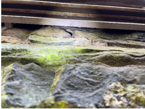
Photograph 6: Narrow gap, ranging from approximately 1 cm to 4 cm, between the timber track of the sliding door and the stone elevation.
