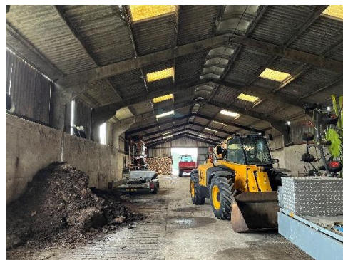
Photograph 16: View of the internal space of the corrugated/timber barn.
